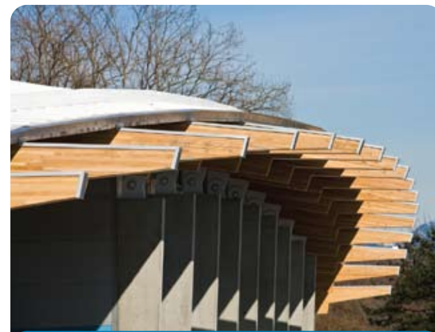
The elegant new Trout Lake rink, first phase of this community recreation complex's renewal, showcases BC wood throughout including downed timbers from Stanley Park.
