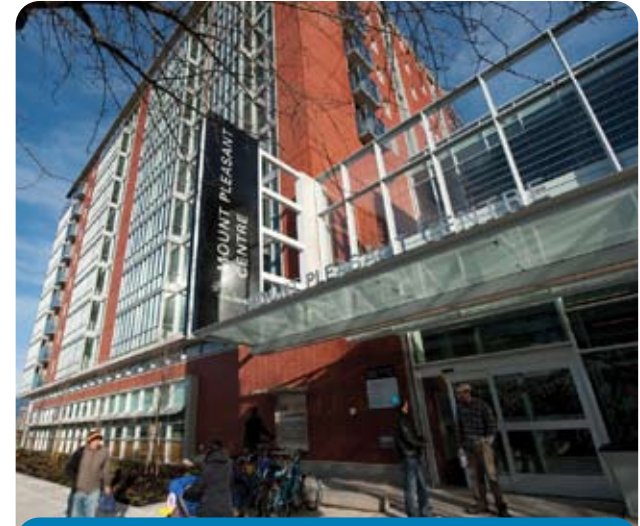
The Mt. Pleasant Community Centre is at the heart of the exciting new multi-service facility at 1 Kingsway.
