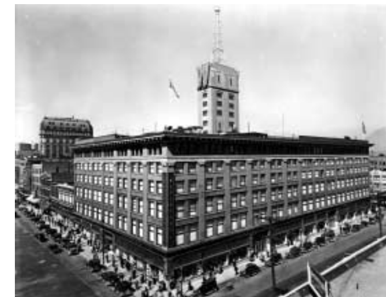
LOOKING NORTHWEST AT ABBOTT AND HASTINGS
