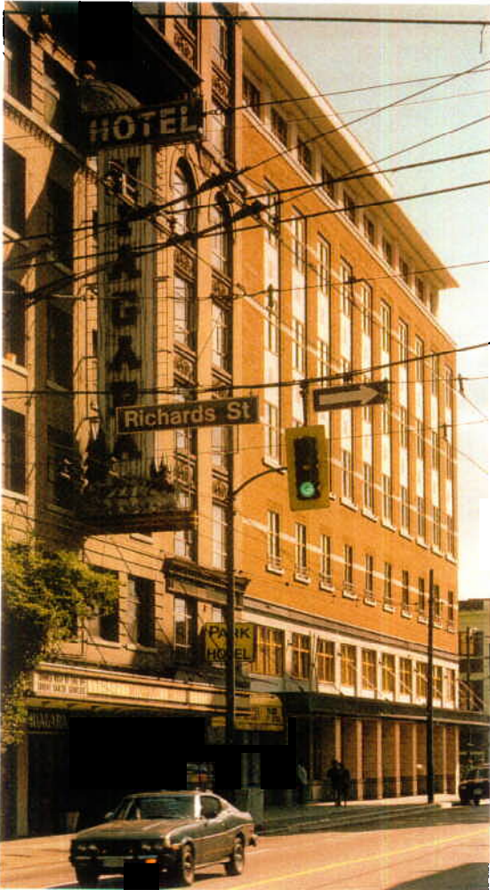
Pender Street facade continues historic streetwell
