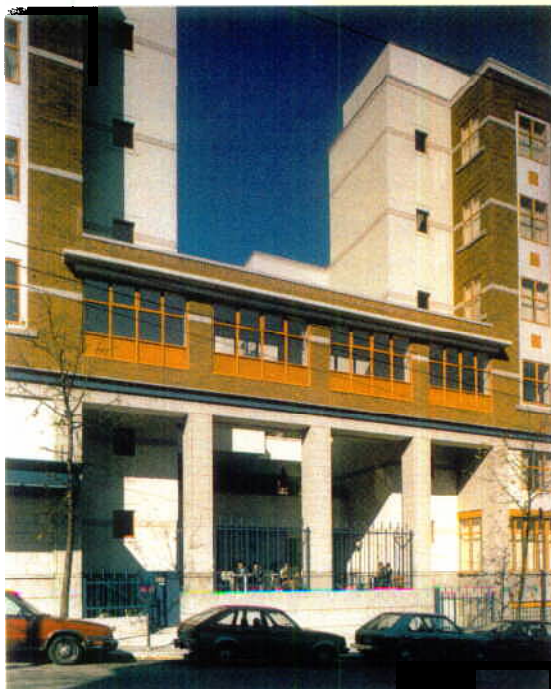
Homer Street courtyard and bridge
