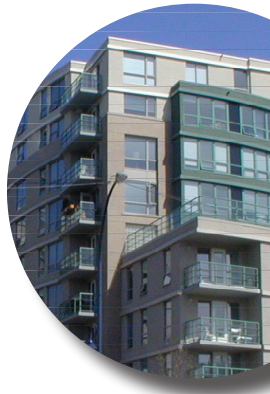
Quayside 1010 Pacific Boulevard 93 units (1999)
