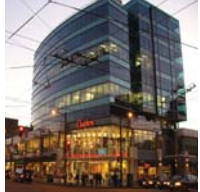
Ensuring adequate job space
