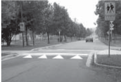
Speed table: raised pedestrian crossing to slow cars
