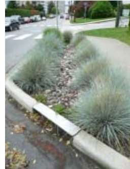
Permeable infiltration landscaping with rocks, not with standing water
