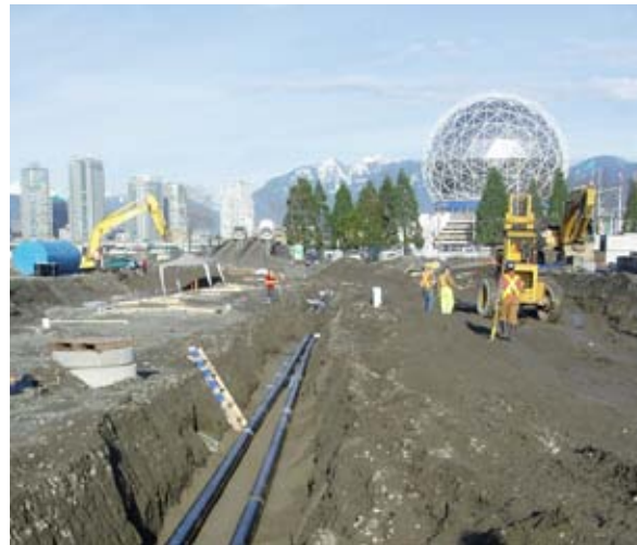
Olympic Village NEU Distribution Pipe Installation Underway
