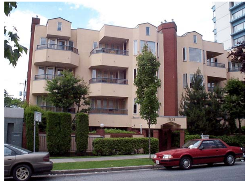
Apartment Building to the south of 911 Denman
