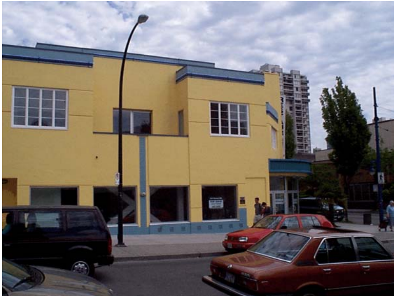
Barclay Street Facade
