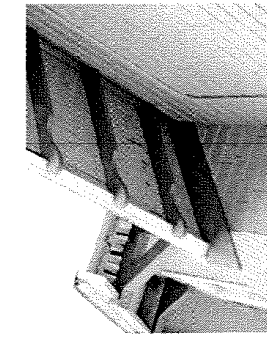
PHOTO VIEW- HIGH ROOF SCROLL CUT RAFTERS & TRIANGULAR ROOF BRICKETS
