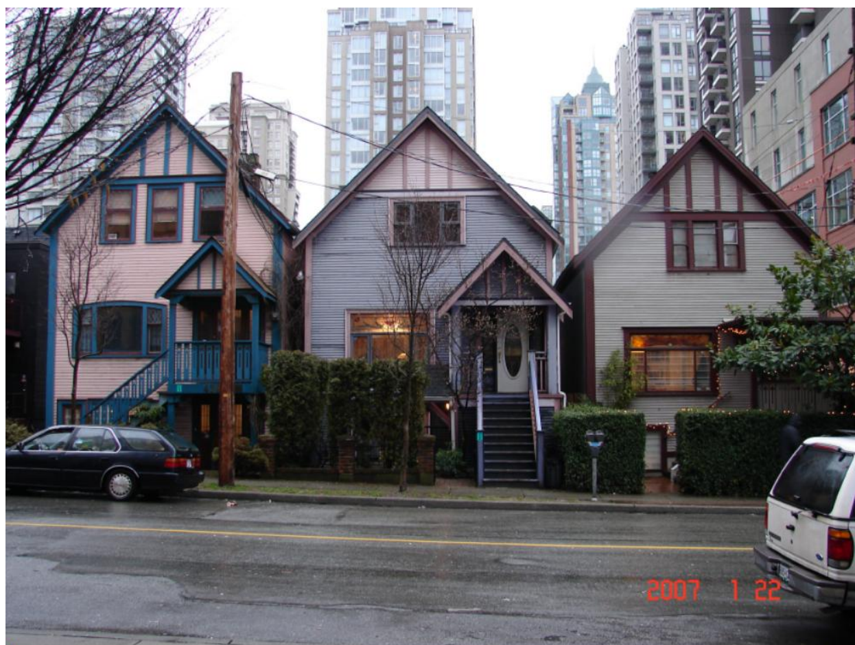
Photo 1: The Helmcken Street Houses Looking North
