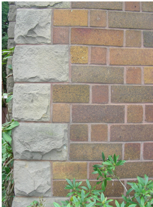
Photo 4: Close up of Masonry Detail
