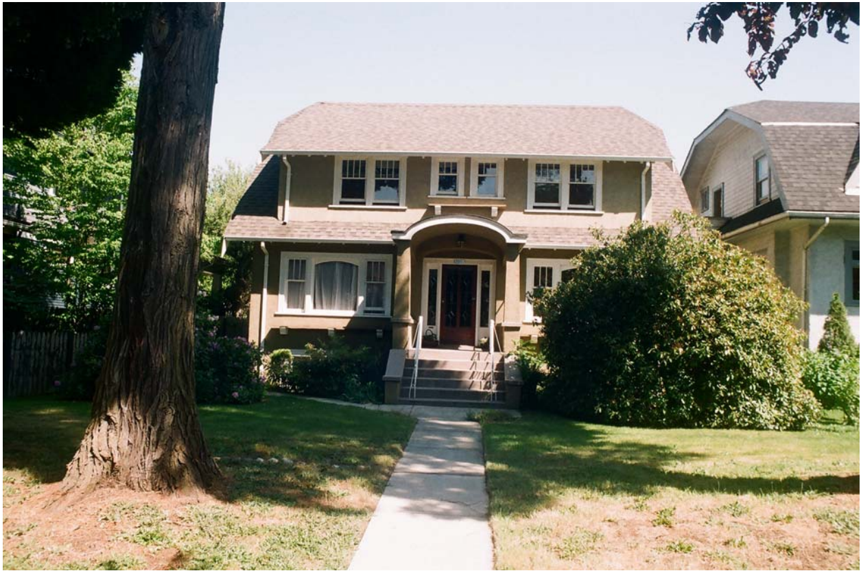
Photo 3: View of 'The Sanderson House' directly from the South
