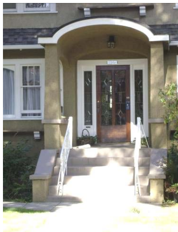
Photo 2: Close up of the Covered Portico
