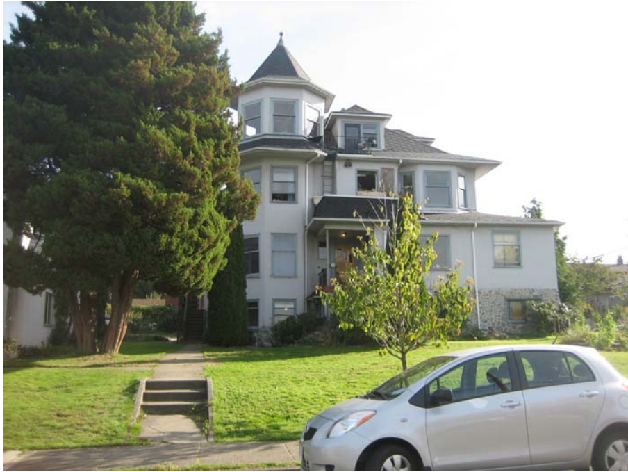
Photo 1 : West side of 'The Jeffs Residence' (2011)
