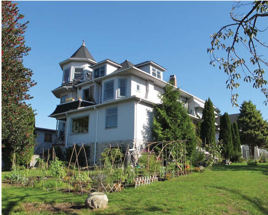
Photo 2 : South-west corner of 'The Jeffs Residence' (2011)
