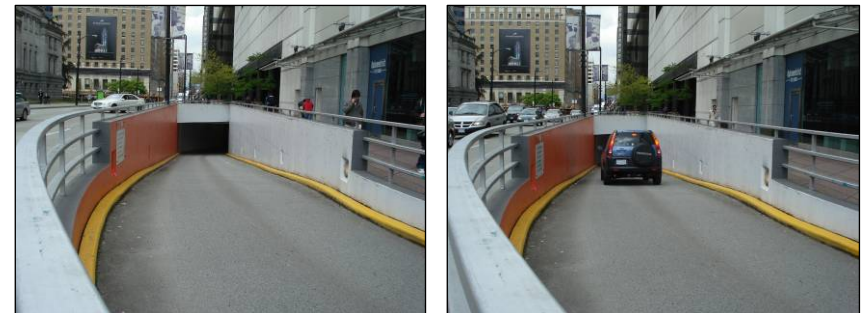
Figure 2.7: Views of Robson Street Entrance
