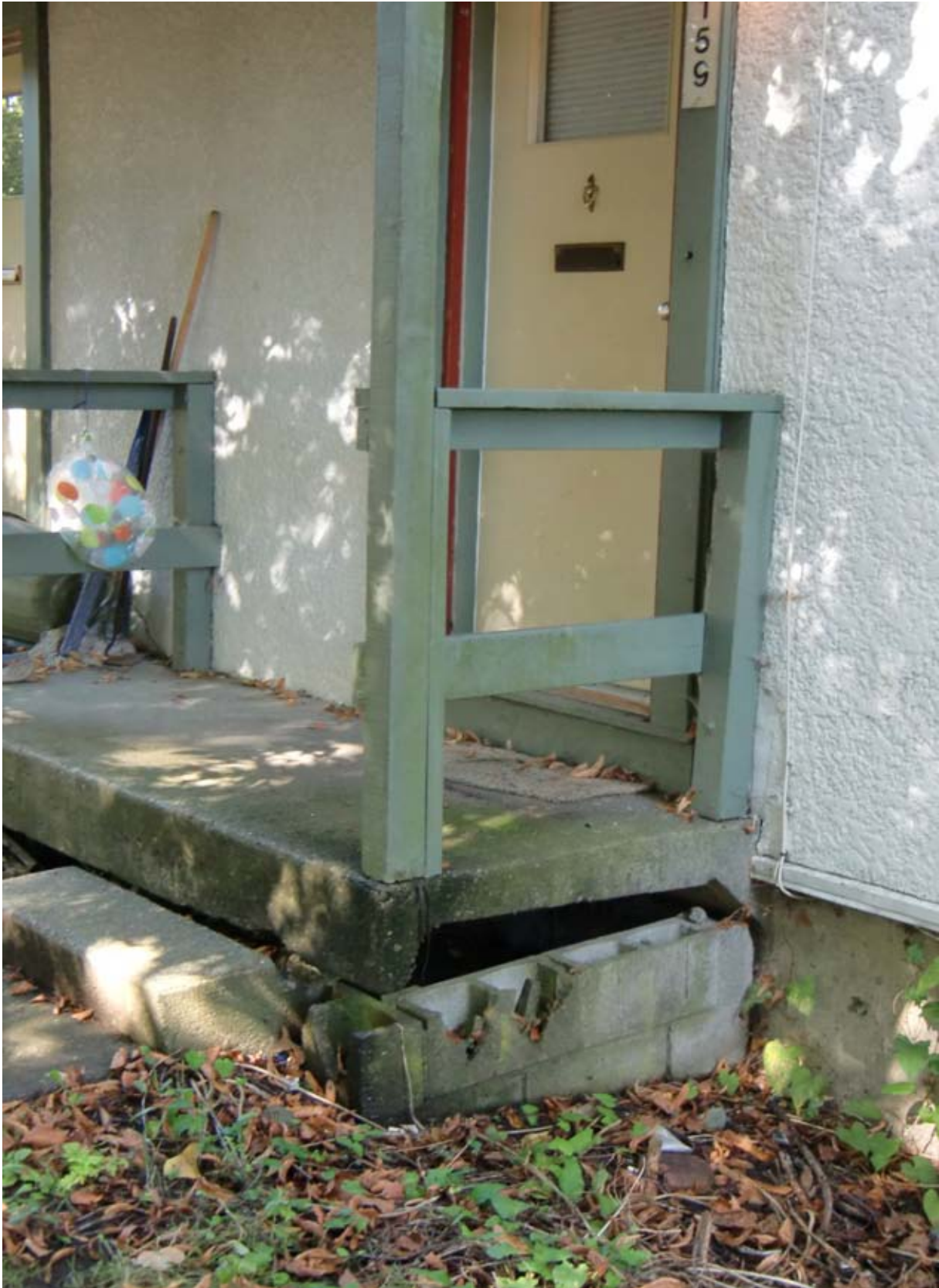
The slabs are functional but the adjacent soils have settled and the steps in general are unsafe. (Refer to Section 7.0)
