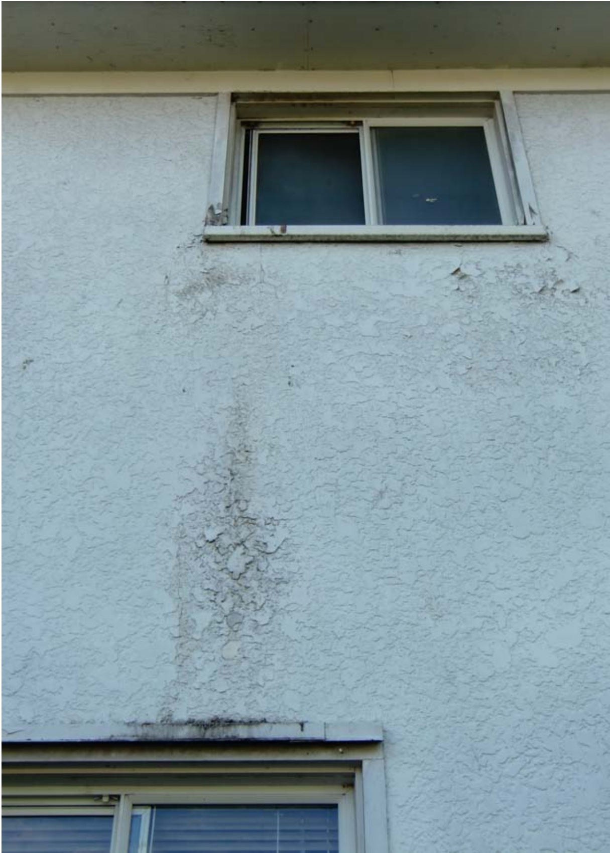
Peeling paint and stained stucco below the bathrooms (Refer to Section 6.0)
