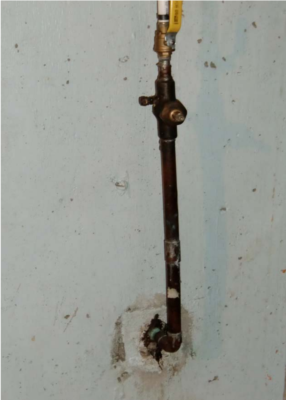
There is no pressure reducing valves at main water services (Refer to Section 2.0)
