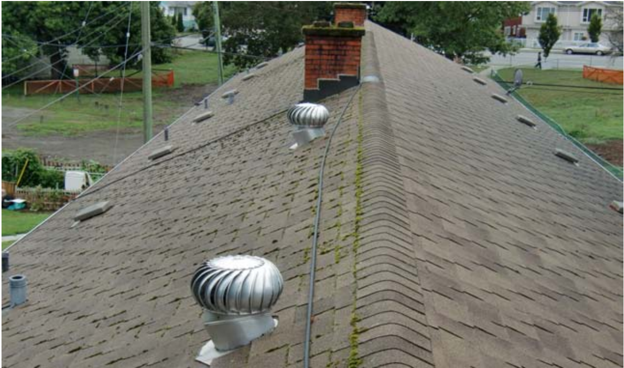
The sloped (approximately 10/12 pitch) roofing appears to be a single layer of interlocking composition shingles installed over a tar felt underlay on solid shiplap (board) sheathing. (Refer to Section 8.0)
