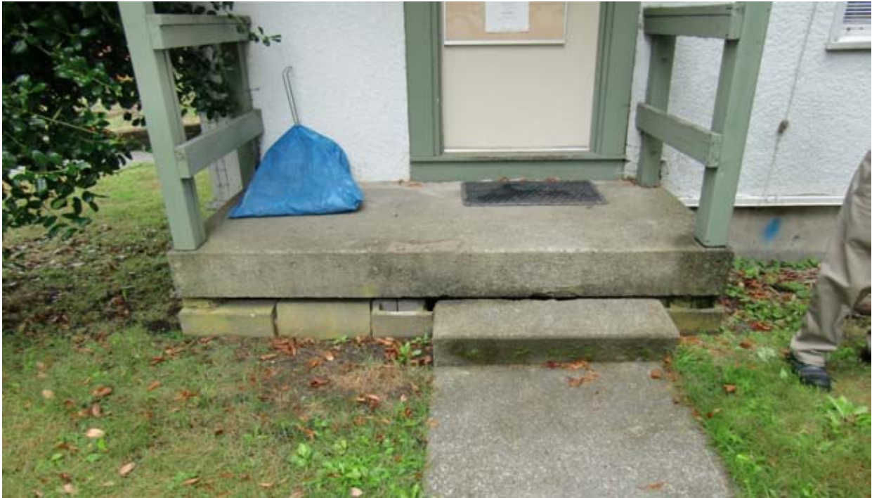
Both the metal and wood guards are also technically unsafe. (Refer to Section 7.0)
