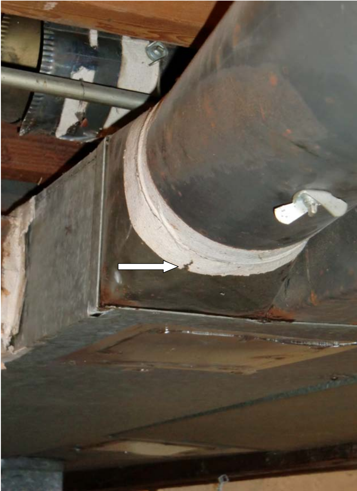
Damaged white duct tape may contain asbestos (Refer to Section 3.0)
