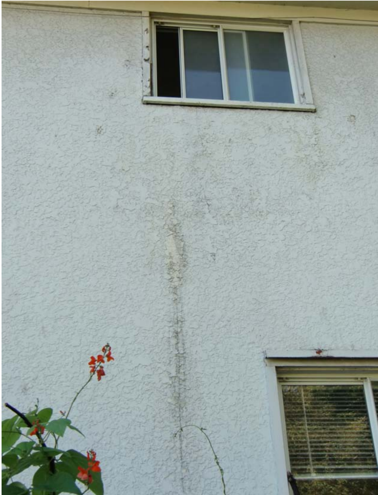
Peeling paint and stained stucco below the bathrooms (Refer to Section 6.0)
