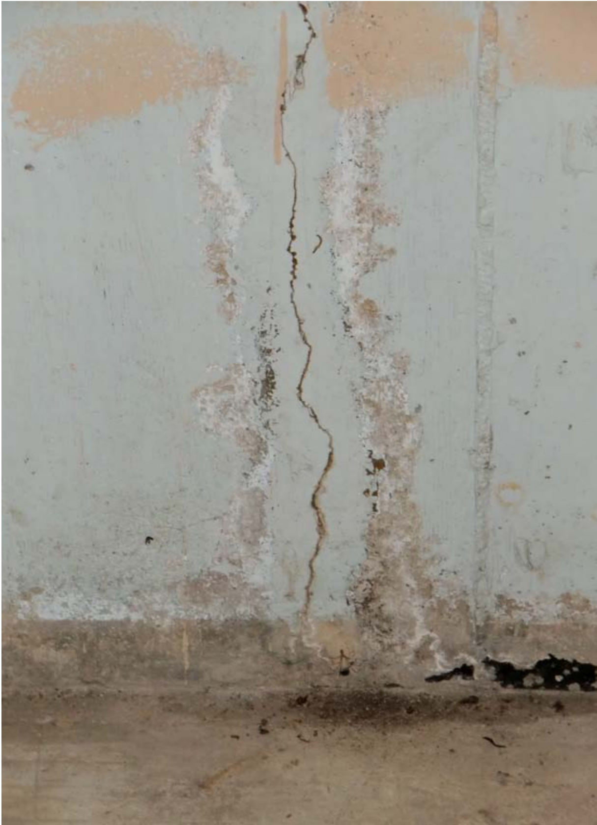
Efflorescence/staining indicating past ground water penetration in basement. (Refer to Section 10.0)
