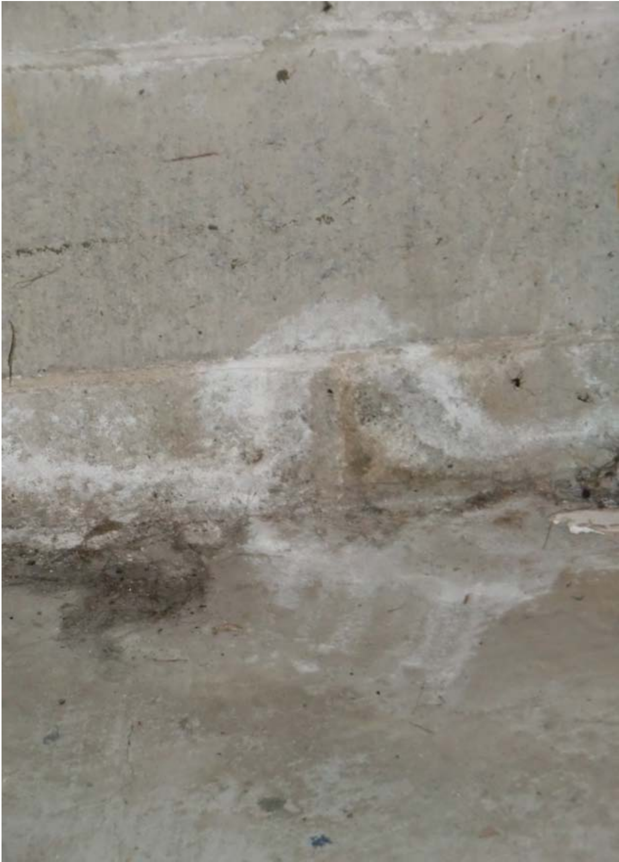
Efflorescence/staining at bottom of CMU wall. (Refer to Section 10.0)
