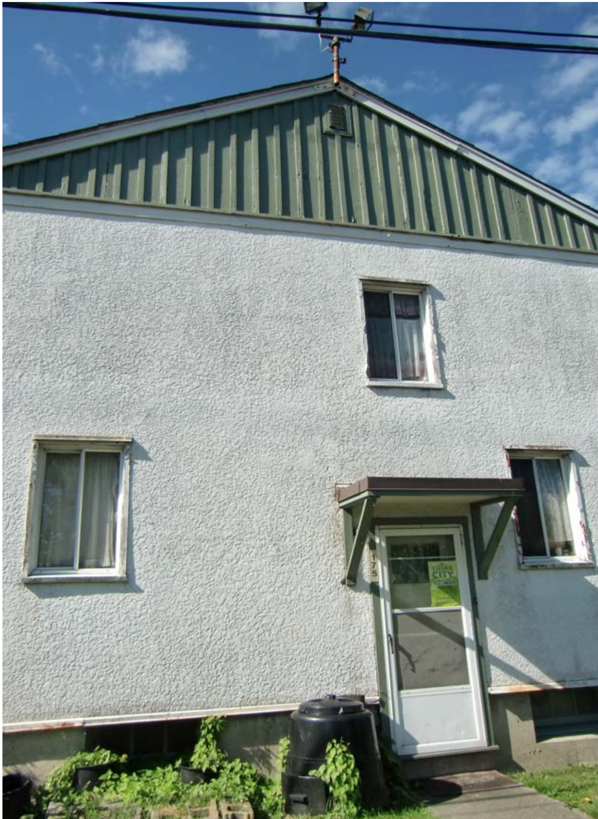
Warping and splitting visible to the wood vertical channel siding at the gable ends. (Refer to Section 6.0)
