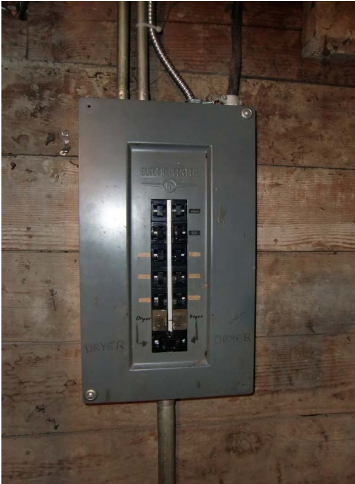
100-amp obsolete Bulldog "pushmatic" electrical panel (Refer to Section 4.0)
