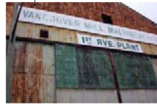
Wilkinson Steel Building
