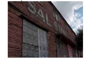
Opsal Steel Building
