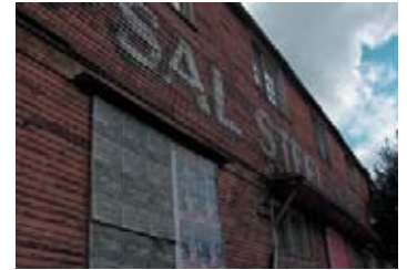
5. Opsal Steel Building
