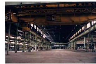
Gantry Crane Gateway Structure
