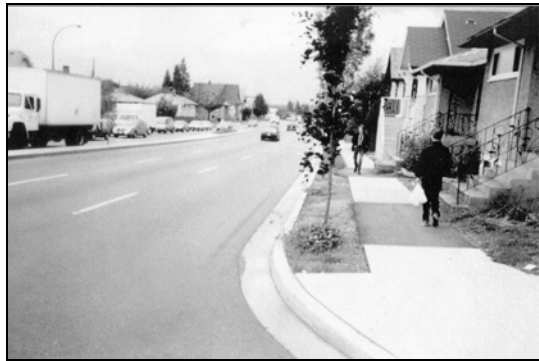
Some front yards have been narrowed where left turn bays have been installed.
