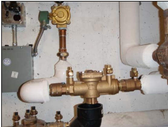
Reduced Pressure Backflow Assembly
