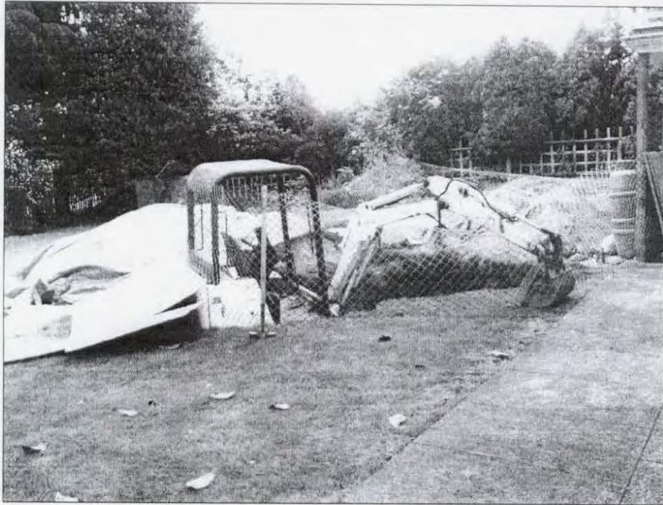
Excavation site's proximity to the building
