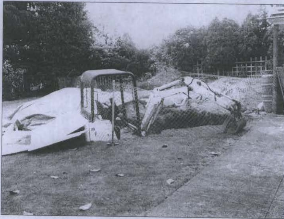
Excavation site's proximity to the building
