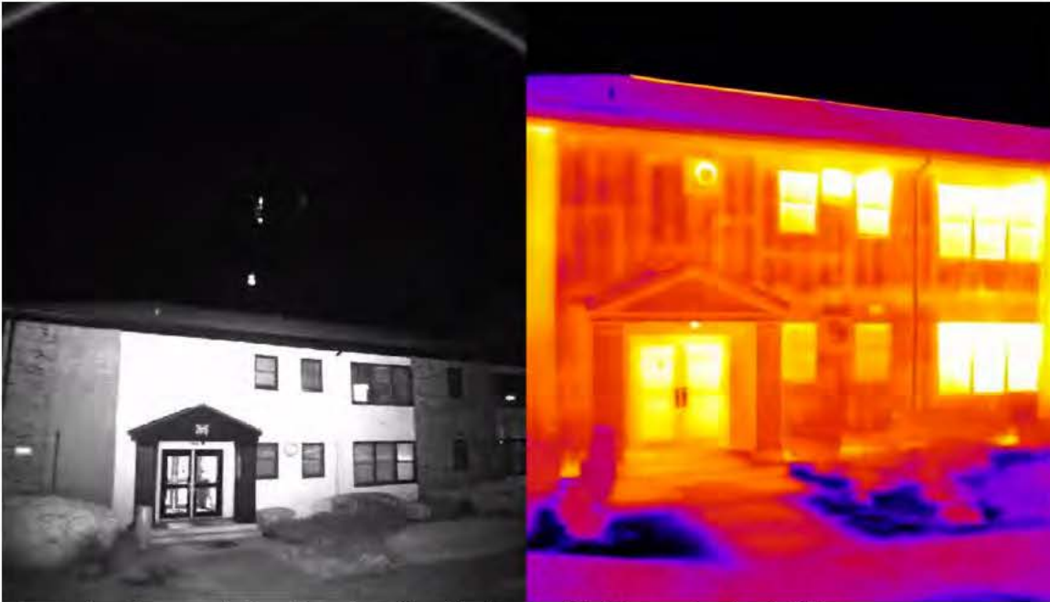
Example of a poorly insulated wall, with thermal bridges clearly visible.
