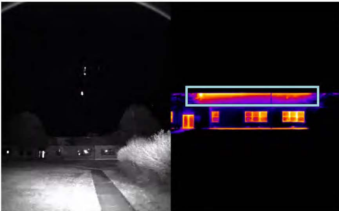
Example of a poorly insulated roof.
