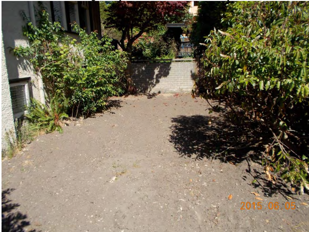
The excavation was backfilled with the onsite clean soils and 2 truckloads of topsoil.
