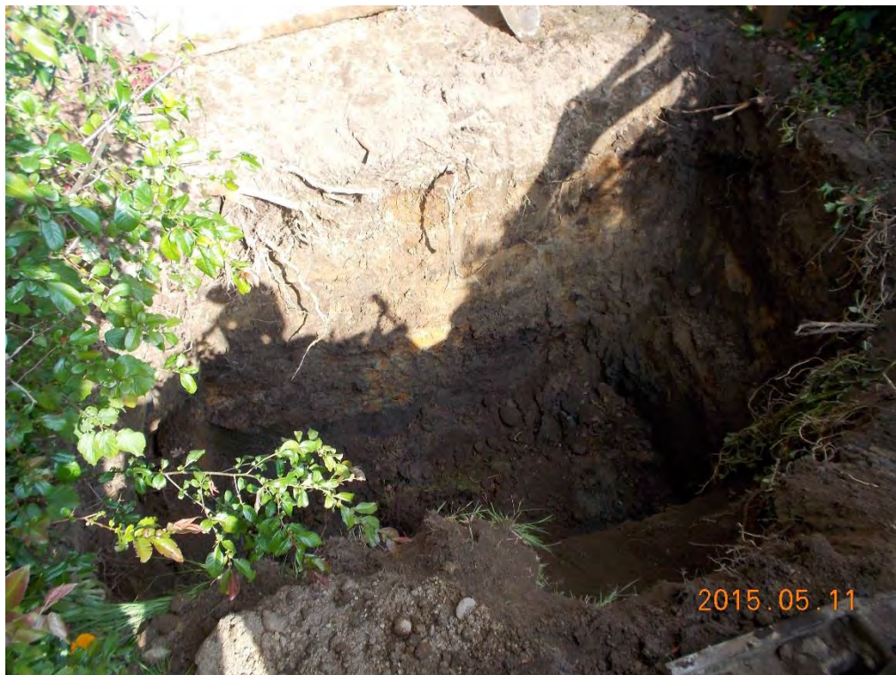
Ventus personnel obtained soils samples May 11, 2015. The base of excavation failed RL standards and all four sidewall samples passed RL standards.
