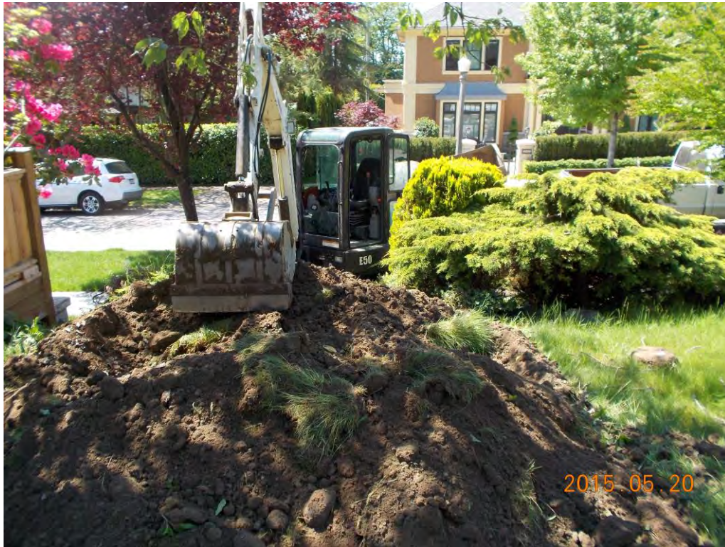
12.01 tonnes of contaminated soils was trucked to Ecowaste Industries located at 10991 Shellbridge Way #200, Richmond on May 21, 2015.
