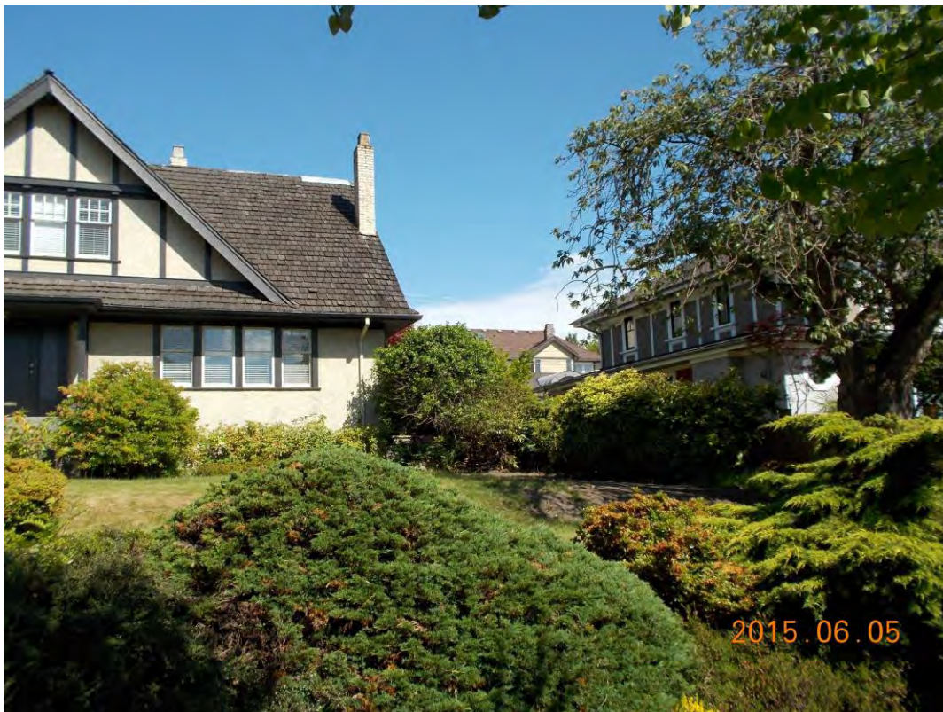
The completed project June 5, 2015.
