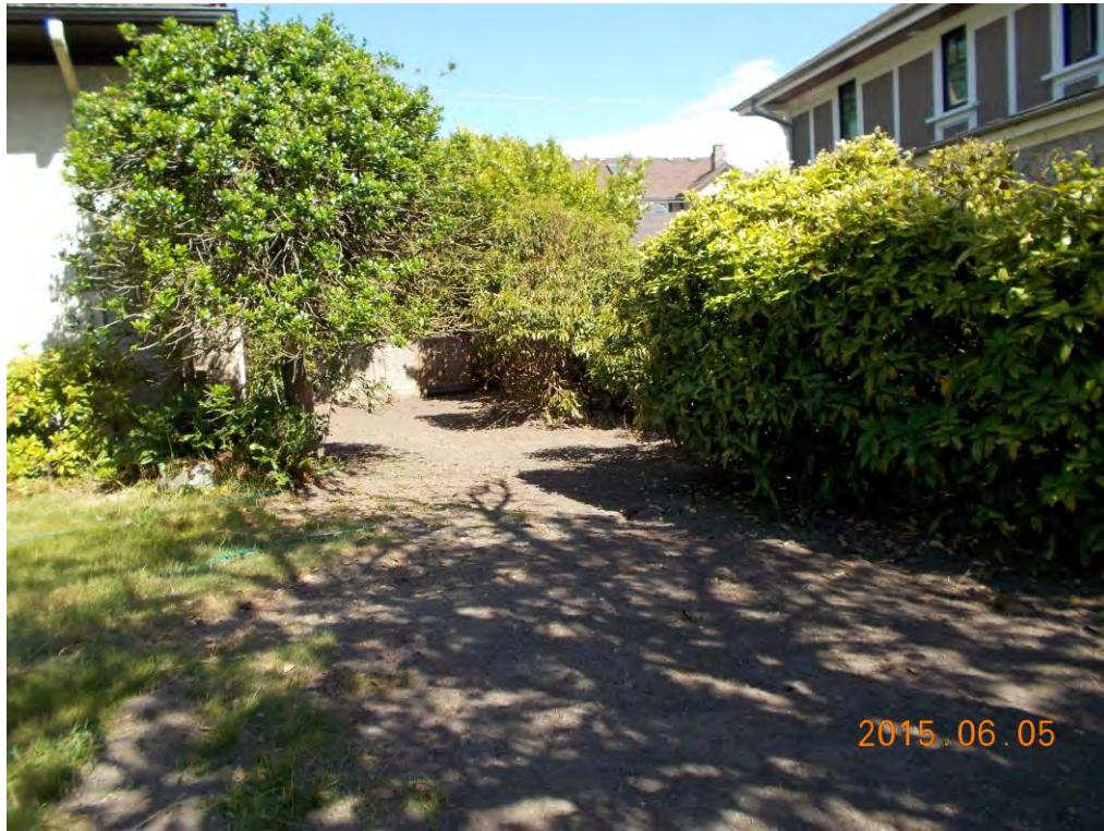
Looking east at the former UST area, the project is completed.
