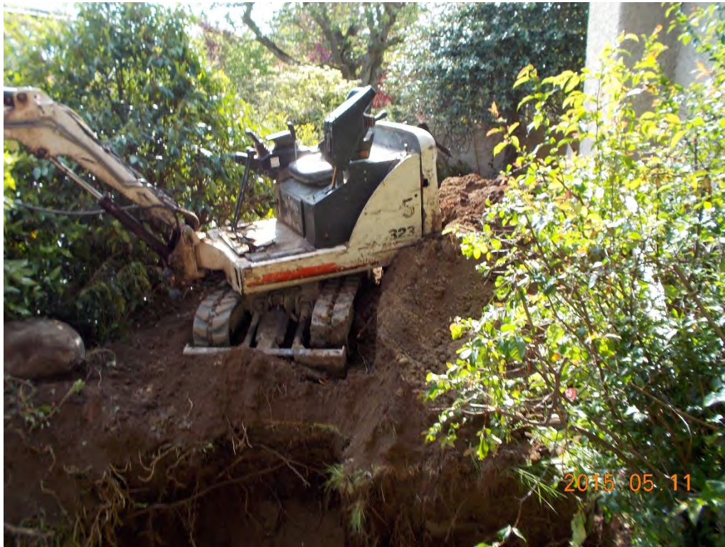
The UST was located south of the southwest corner of the house onsite.
