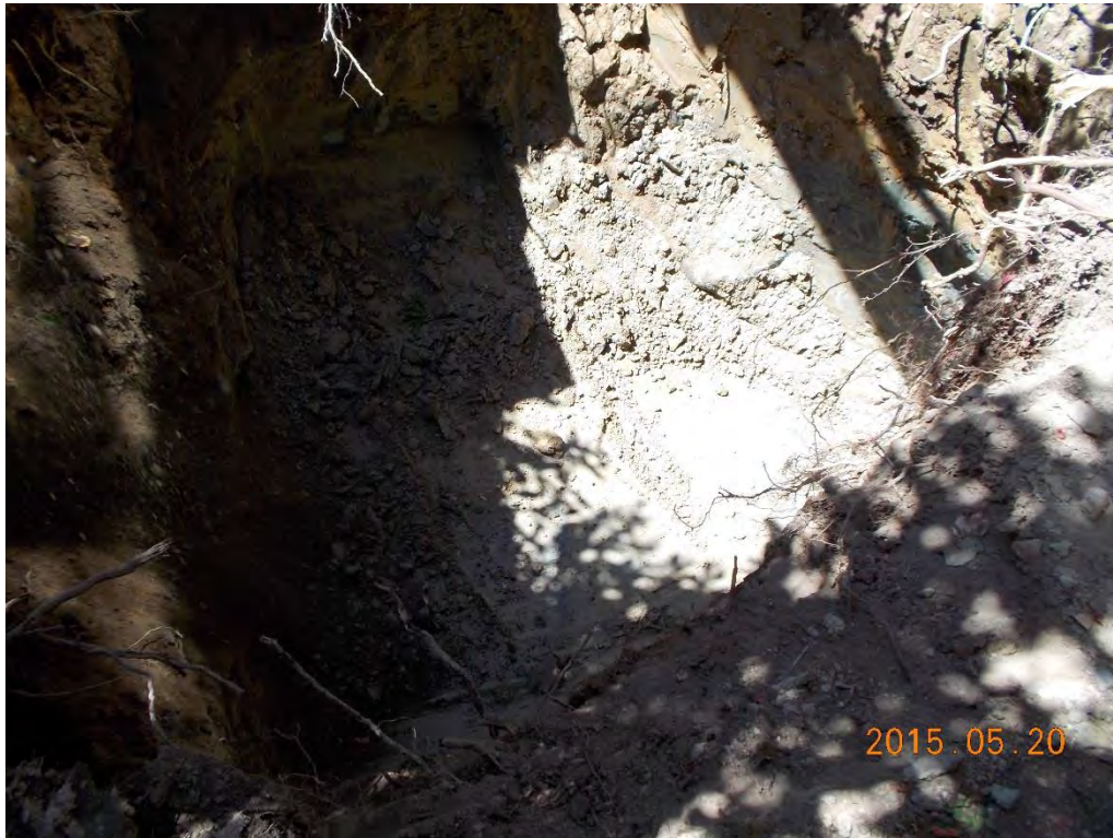
Looking into the excavation after excavation of the contaminated soils May 20, 2015.
