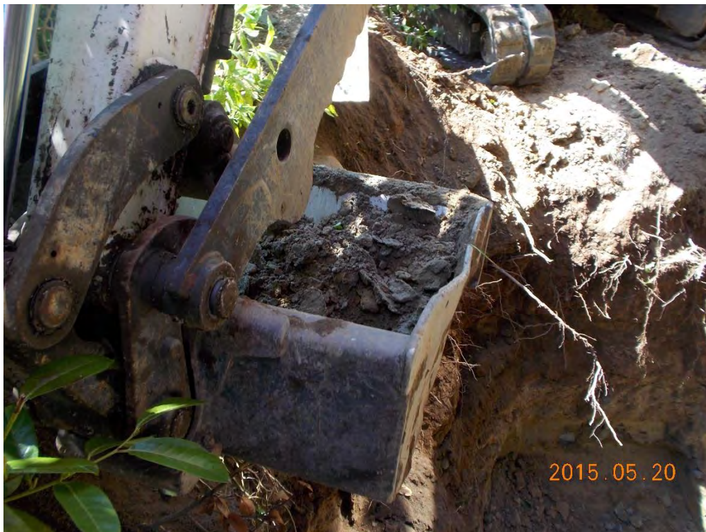
A base of excavation closure soil sample was obtained May 20, 2015, it passed RL standards.
