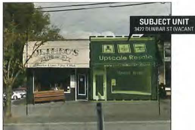
EXISTING STOREFRONT VIEW EASTWARD VIEW
