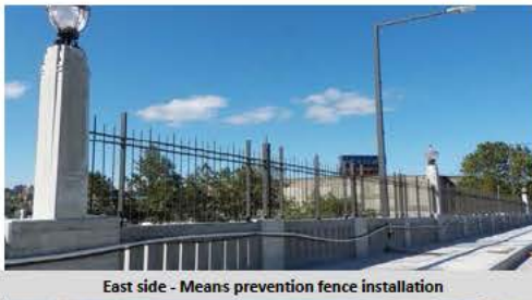
East side - Means prevention fence installation
