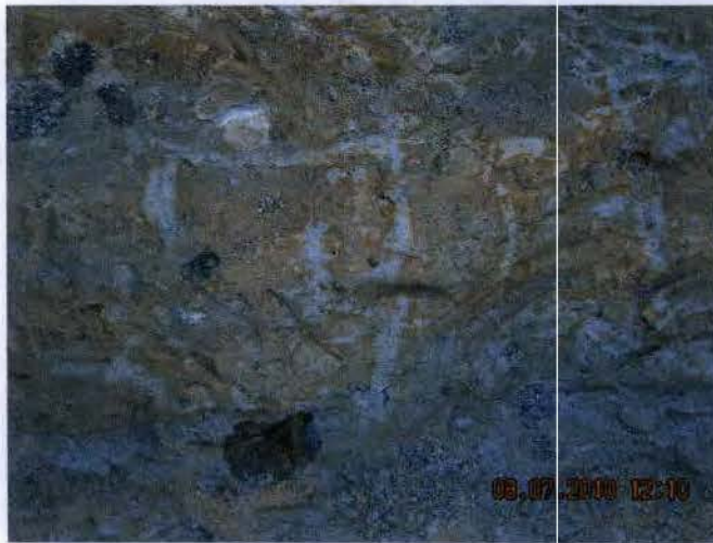
Photo 9 - Impacted soil veins on excavation wall
