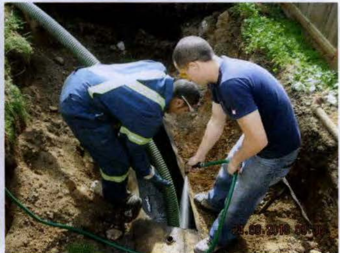
Photo 4 - Rinsing the tank
