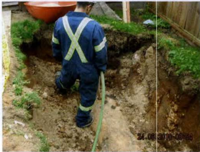
Photo 3 – Pumping out the tank
