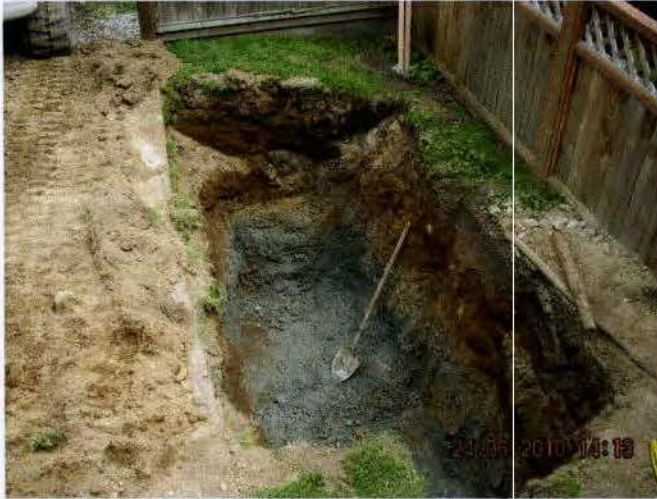
Photo 7 - Signs of contamination
