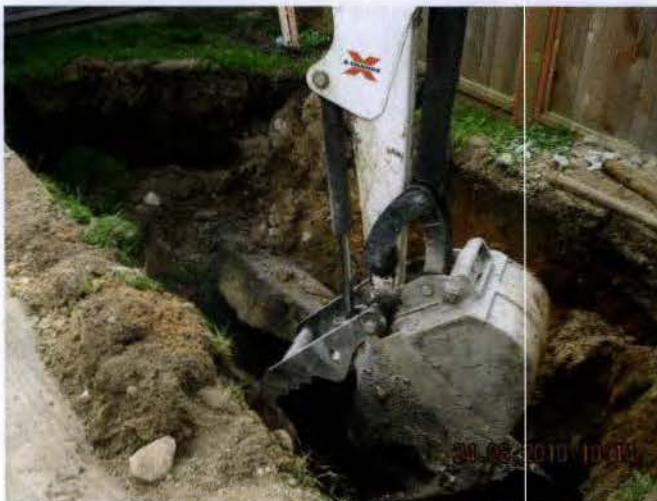
Photo 5 - Extracting the tank
