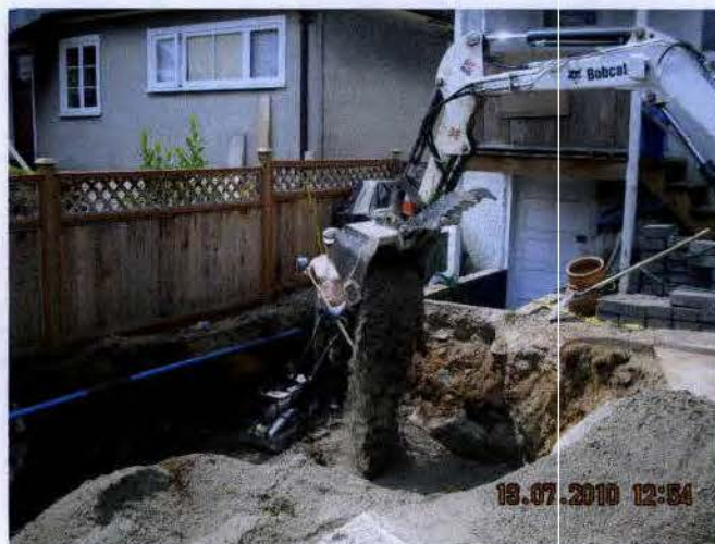
Photo 11 - Backfilling and compacting
