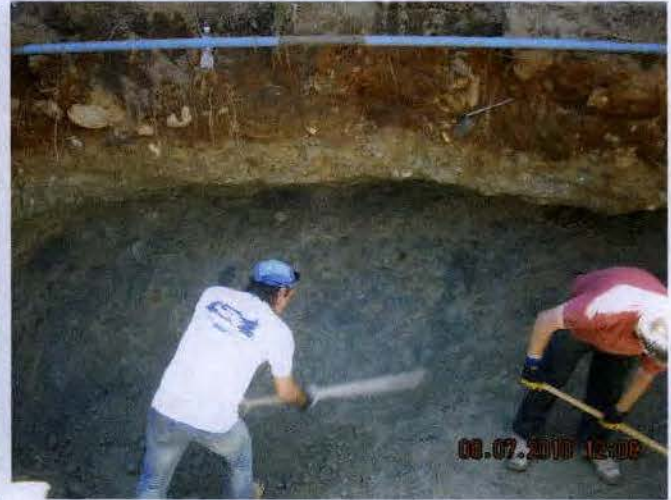
Photo 10 - Hand digging the last remaining impacted soils
