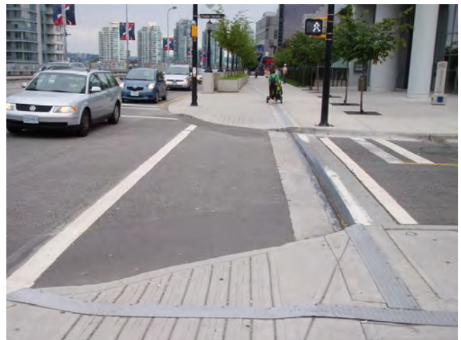
D-8 I-06.jpg Longitudinal joint between deck and sidewalk structure at west approach.
