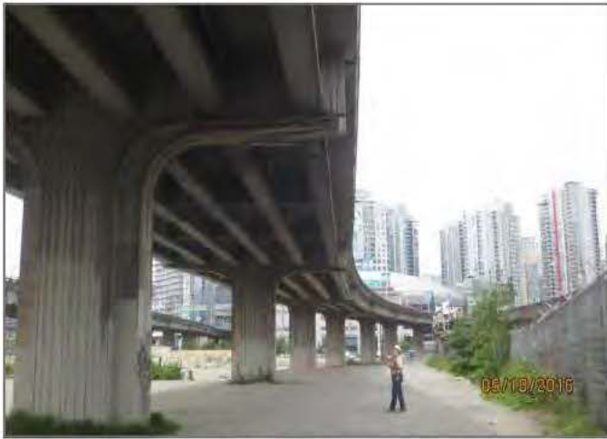
G7. General view looking west from Pier D8.
