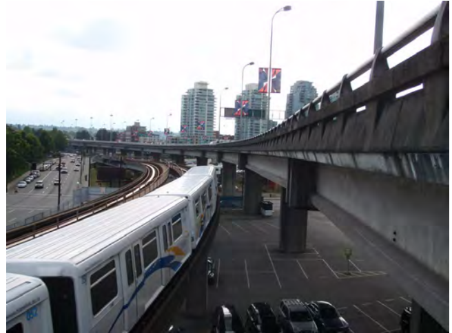
D-8 I-02.jpg North elevation, looking east.
