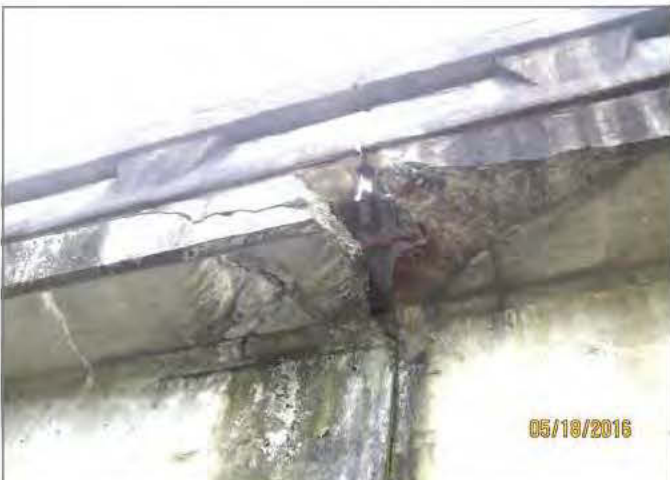
D5. Deck overhang spall on on-ramp approach.
