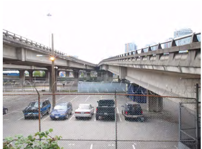
D-8 I-04.jpg Looking west from east abutment at main structure and ramp.
