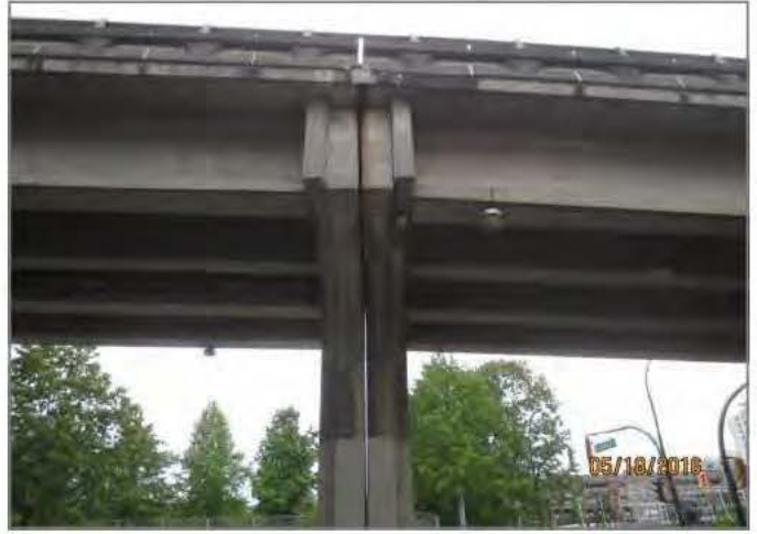
G8. Gap between piers at expansion joint; Pier DM5 shown.
