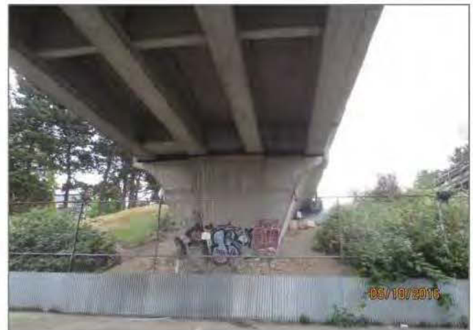
G4. General view of east abutment at D2.
