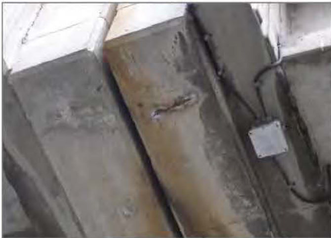
D3. Pier cap soffit spall with exposed rebar at Pier DM5.
