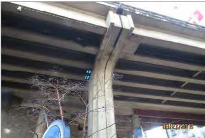
P7. Pier cap joint seal installed at Rogers Arena Plaza.
