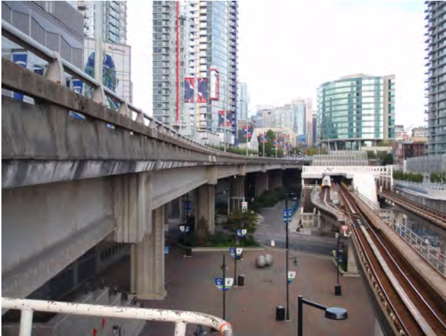
D-8 I-01.jpg North elevation looking west.
