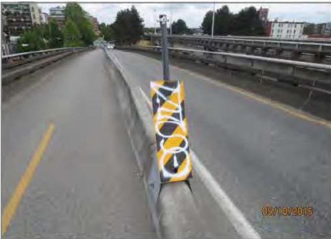
D21. Broken hazard sign at on-ramp bike lane taper.
