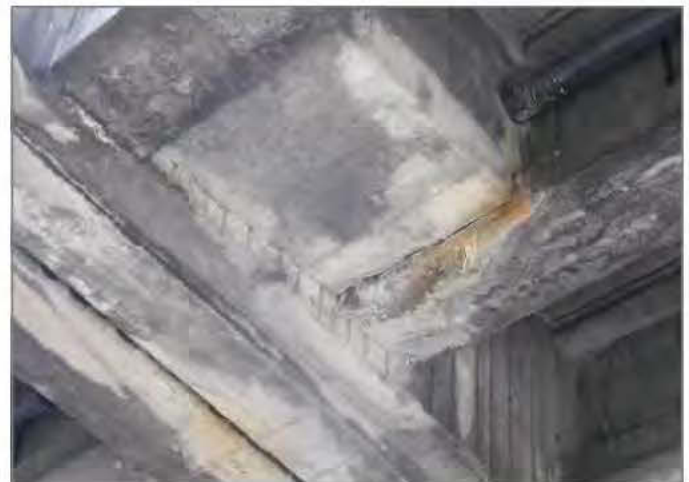
D22. Staining of concrete at base of utility box at Pier D9.
