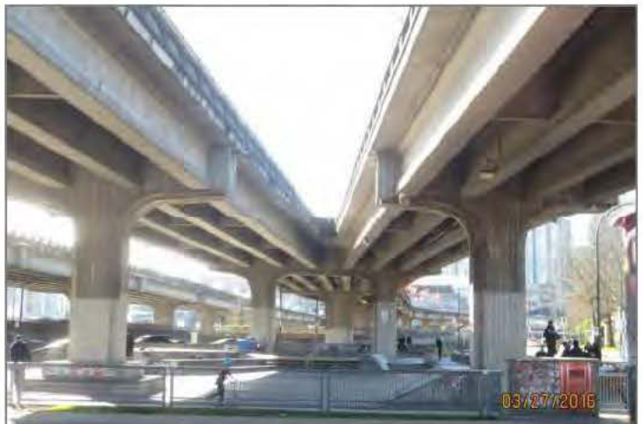
P8. General view of main line (left) and on-ramp (right) junction above the skate park.
