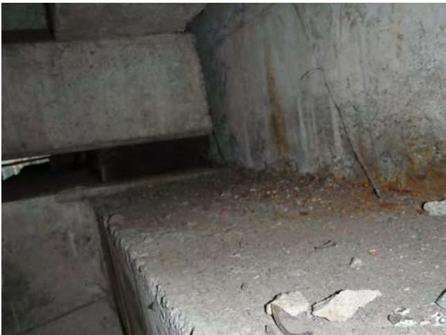
D-8 I-29.jpg Typical bearing at Main Street ramp east abutment.
