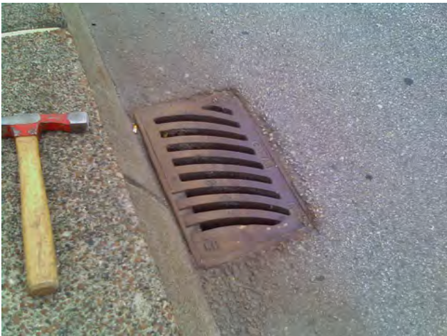
D-8 I-17.jpg Typical catch basin.
