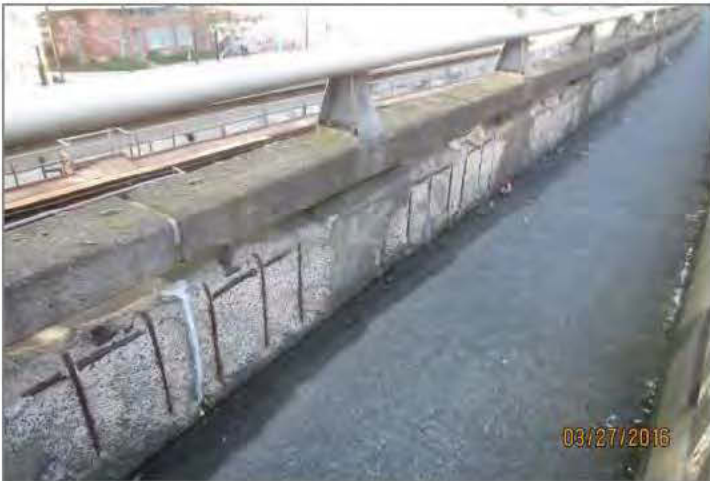
P5. Spalling to outside face of parapet at north sidewalk north of Rogers Arena.
