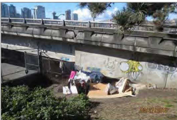
P1. Encampment established at east abutment of on-ramp.
