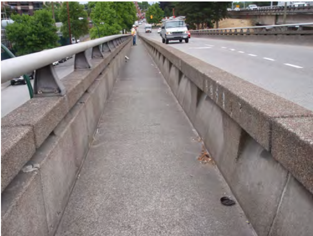
D-8 I-15.jpg Typical sidewalk on ramp.
