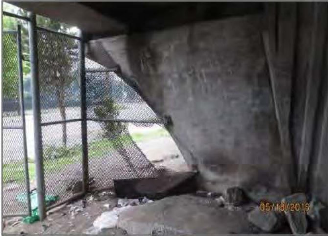
D1. Damaged fencing at on-ramp abutment enclosure (DM2).
