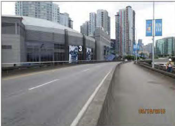
G9. General view of deck looking west from D14.
