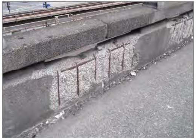
D18. Typical spalls on south face of north parapets.
