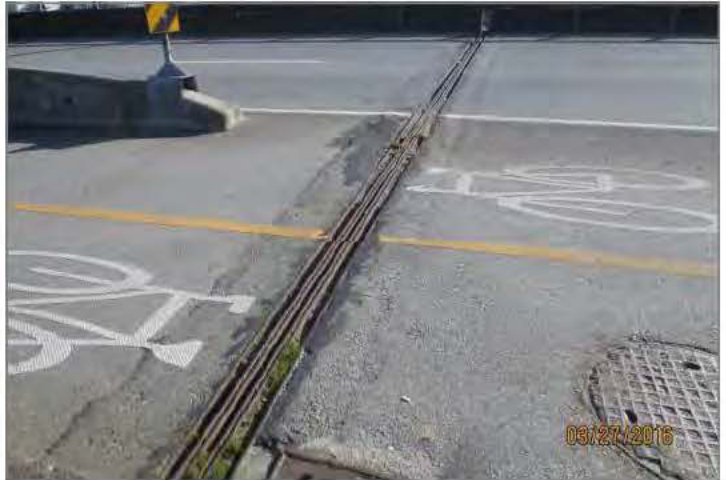
P4. Typical deck joint with large recesses and filled with debris.
