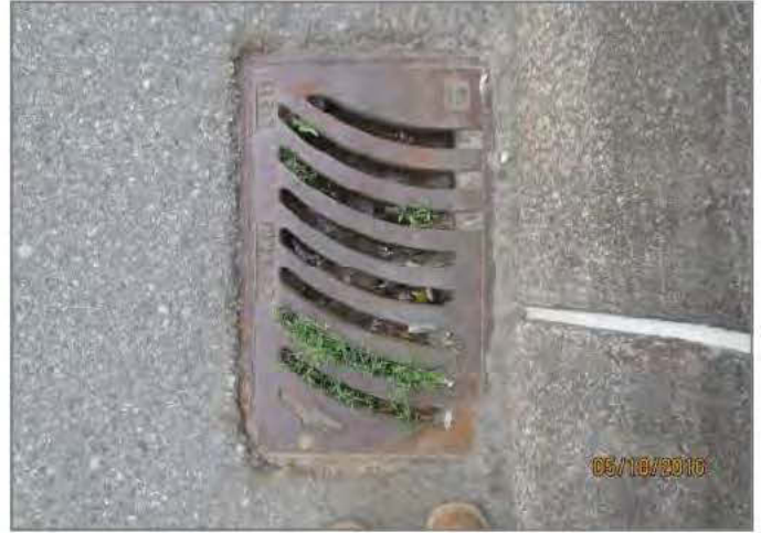
D20. Drain basin filled with debris and vegetation at DM5.
