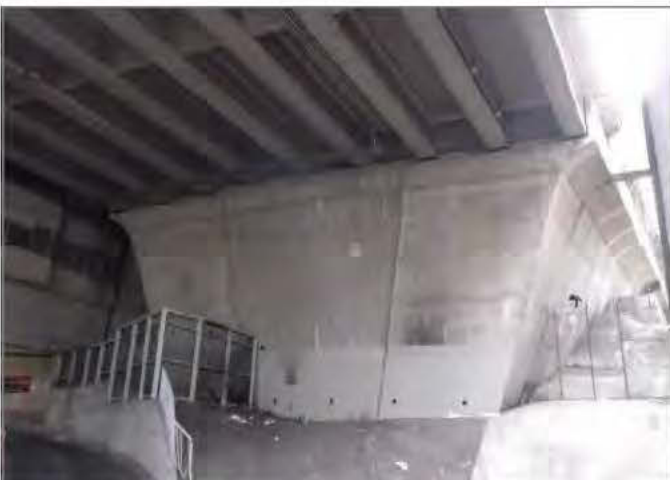
G11. General view of west abutment at D23.
