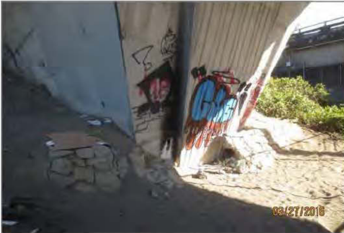
P3. Deficient retaining wall at base of east abutment that is permitting the erosion of soil.
