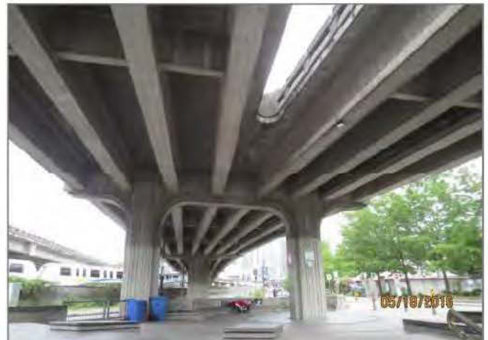
G6. On-ramp junction with mainline at Pier D6.
