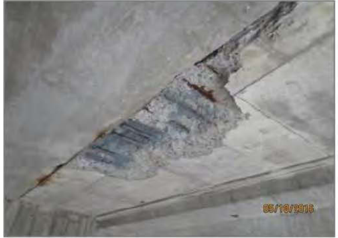
D8. Deck soffit spall with exposed rebar at Pier D6.
