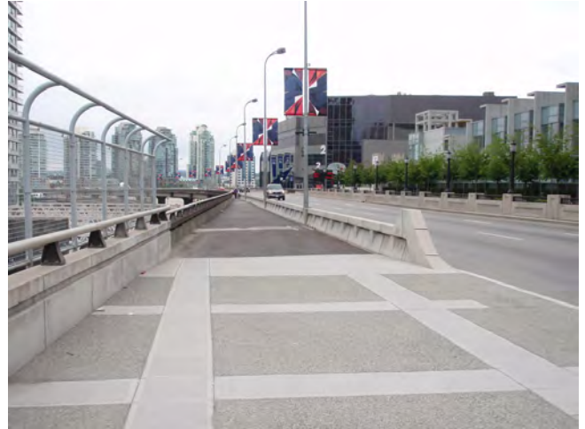
D-8 I-14.jpg Sidewalk flair and replacment bridge rail in west approach.
