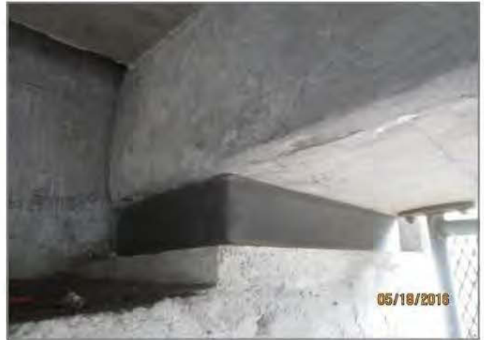
G2. Typical bearing condition at on-ramp abutment (DM2).
