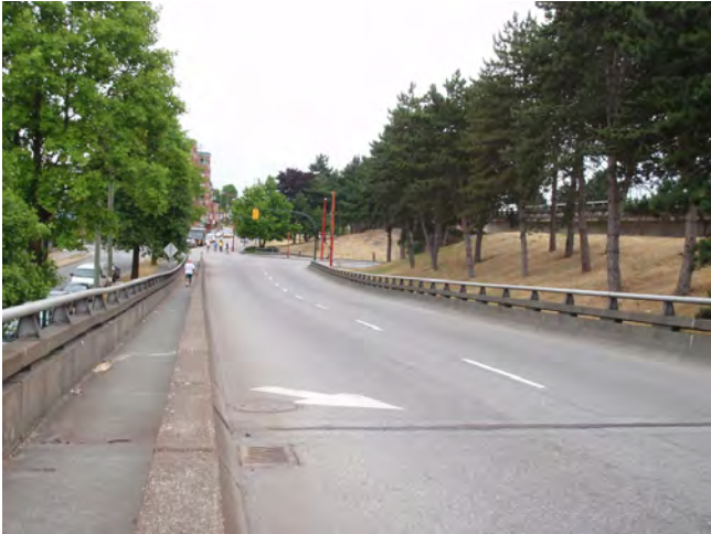
D-8 I-13.jpg Main Street ramp - looking east.
