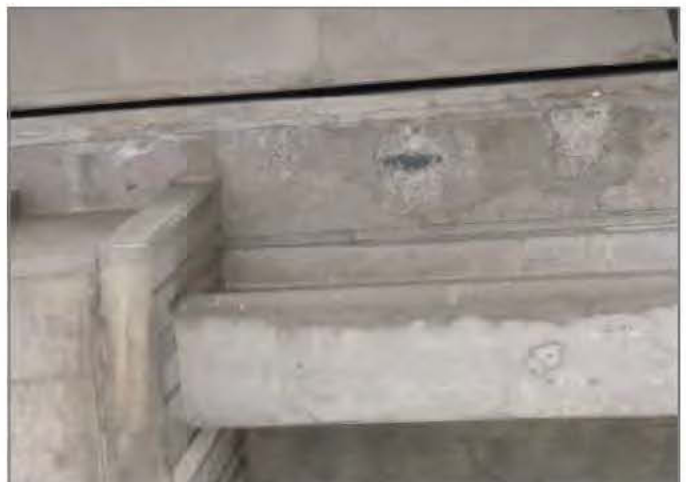
D12. Deck soffit spall at south overhang in span D19-D20.
