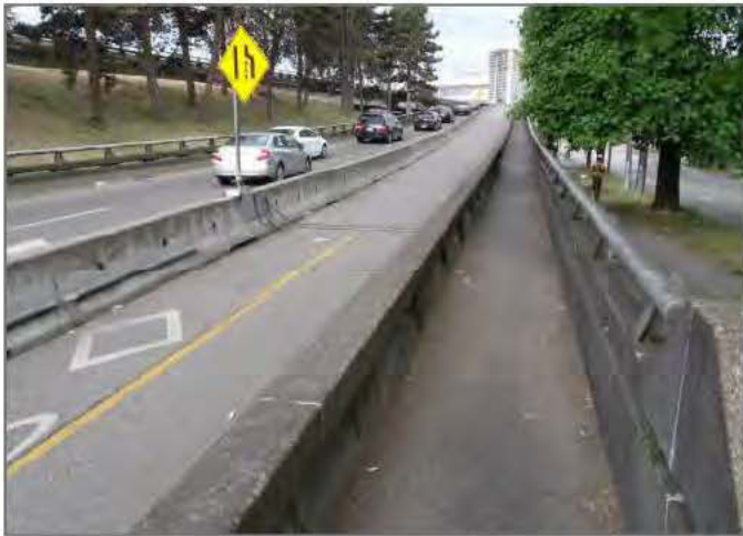
G1. View west along on-ramp approach from Main Street.
