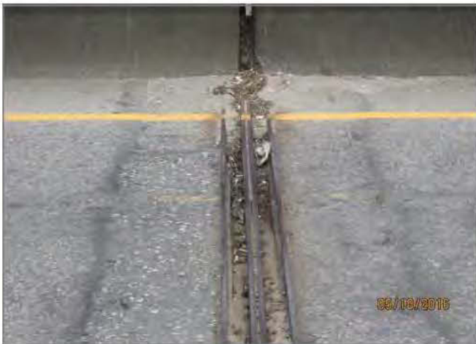
D15. Typical condition of deck joints; torn seals and debris.
