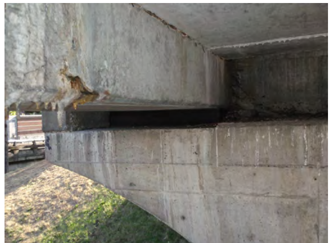
D-8 I-24.jpg Typical abutment bearing.
