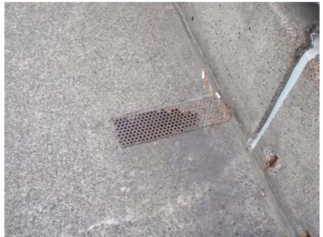
D-8 I-18.jpg Typical sidewalk drain.
