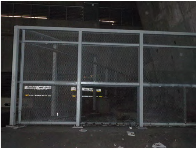
D-8 I-27.jpg Cage around west abutment.
