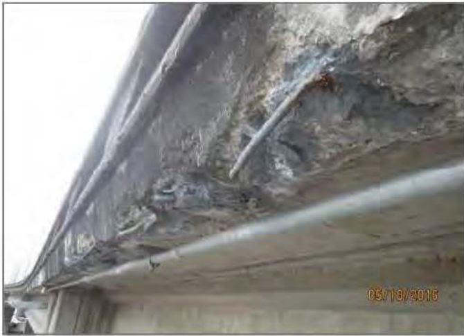
D13. Spalled concrete on north deck overhang span D20-D21.
