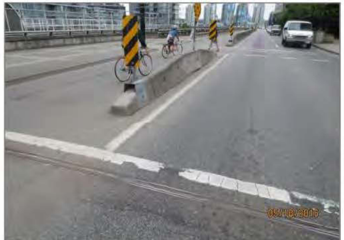
G12. Deck joint at west abutment (D23).
