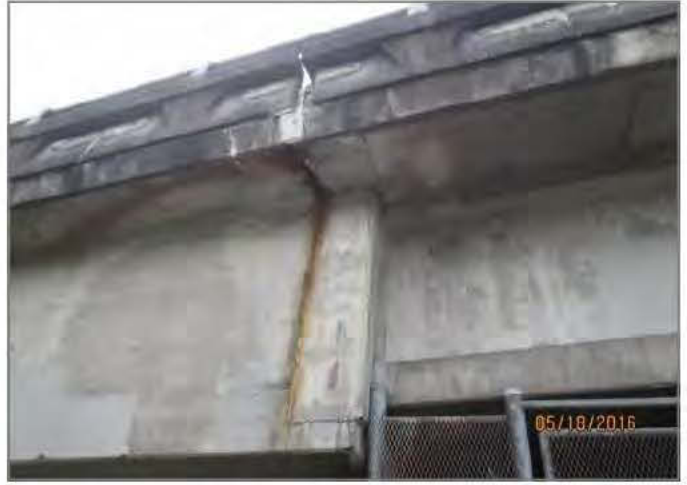
D14. Typical corrosion staining at expansion joint locations.
