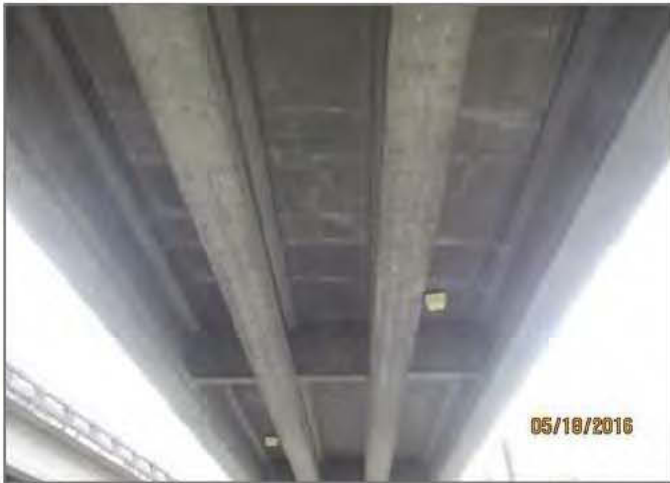
D7. Deck soffit cracks of on-ramp span between DM4-DM5.
