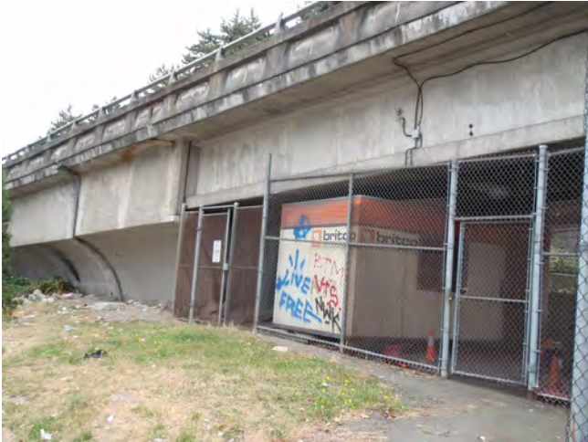
D-8 I-25.jpg Enclosure at east abutment of main street ramp.
