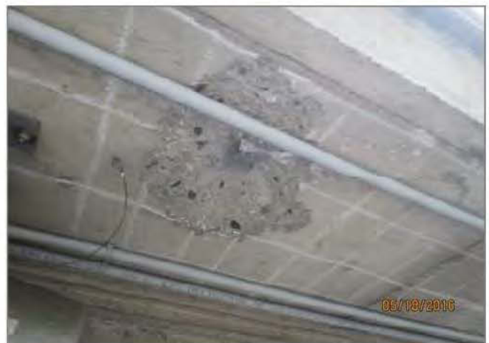
D10. Deck soffit spall at south overhang in span D18-D19.
