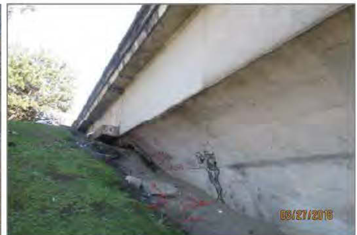
P2. Erosion of soil from north side of east abutment.
