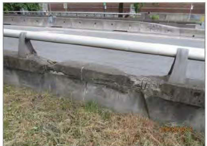
D16. Damage to barrier concrete of on-ramp approach (DM1).
