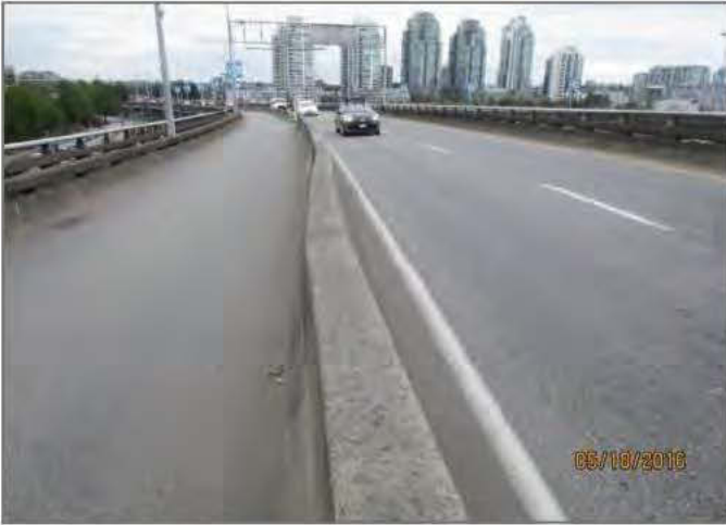
D19. Slight misalignment of traffic barrier near Pier D15.
