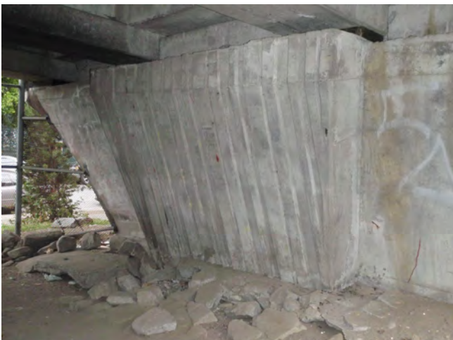
D-8 I-23.jpg Main Street ramp, east abutment (DM2).
