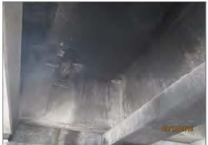
D6. Staining of deck soffit from fire at on-ramp abutment.
