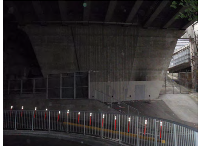
D-8 I-26.jpg West abutment.
