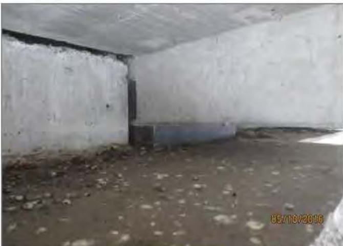
G5. Typical bearing condition at east abutment (D2).
