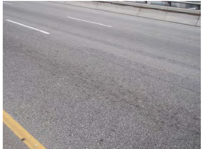
D-8 I-16.jpg Typical wearing surface.
