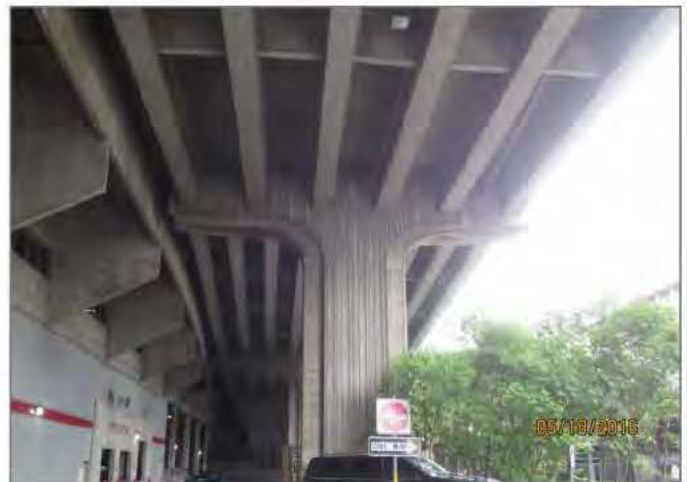
G10. East face of Pier D21 north of the Costco building.
