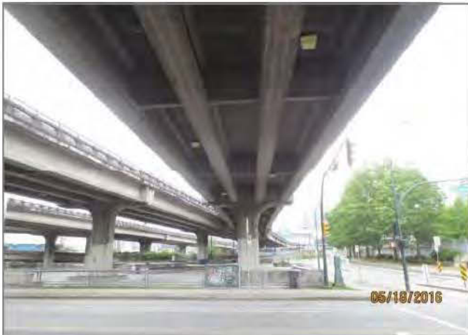
G3. View of on-ramp span DM4-DM5 over Quebec St.
