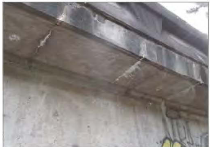
D4. Cracks on deck overhang along on-ramp approach.
