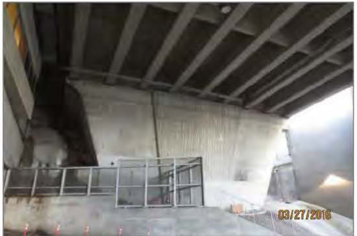
P6. General view of west abutment.
