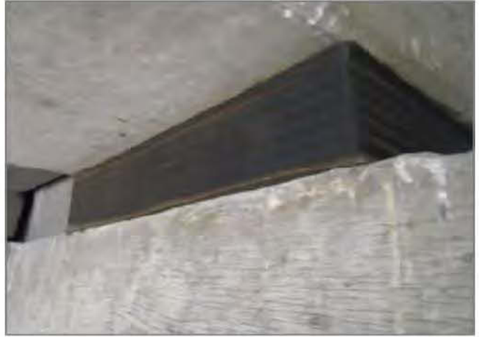
D2. Slight overhang of bearing pad at west abutment (D23).
