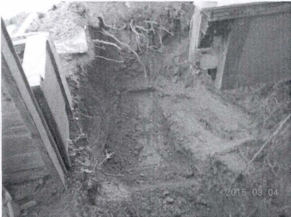
Ventus personnel obtained soils samples March 4, 2015. The base of excavation sample failed RL standards.
