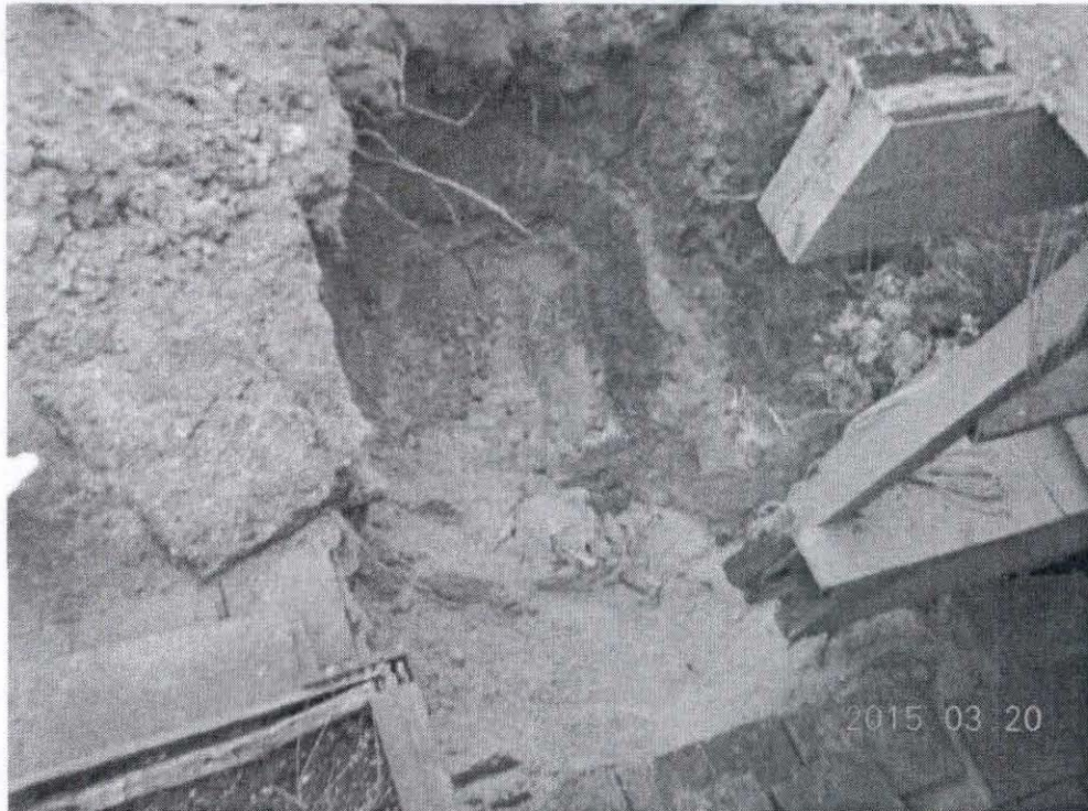
Looking into the excavation after excavation of the contaminated soils March 20, 2015.
