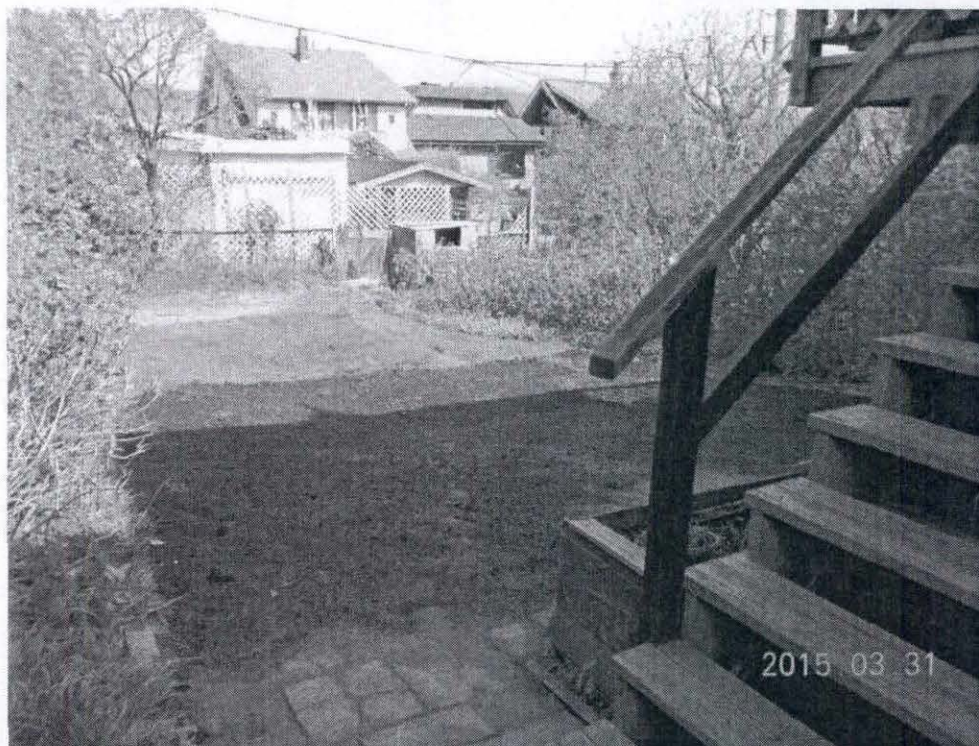
The excavation was backfilled with the onsite clean soils, 7.5 yards of sand and 3.5 yards of topsoil March 30 th , 2015.
