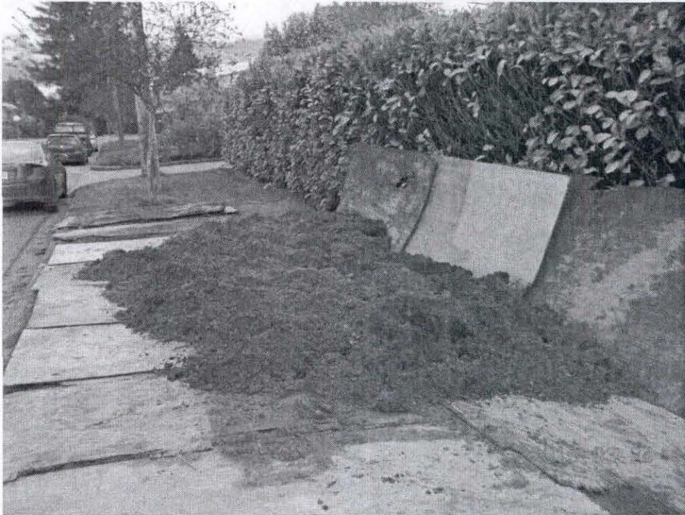
One soils bin of contaminated soils was trucked to Sumas Remediation Services on 4623 Byrne Road in Burnaby March 25th, 2015. These are the contaminated soils.
