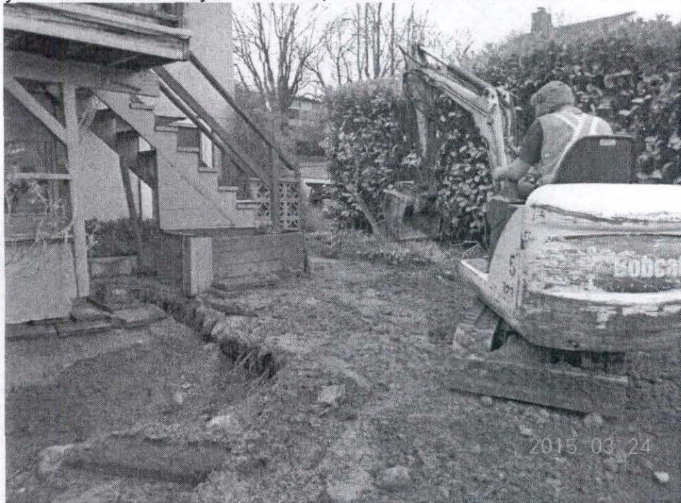
Looking northwest at the former UST area now partially backfilled March 24, 2015.
