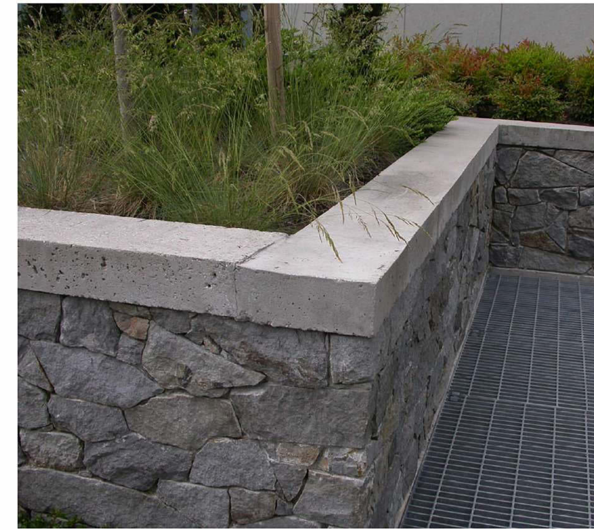
9 STONE CLAD CIP CONCRETE WALL L6.2
