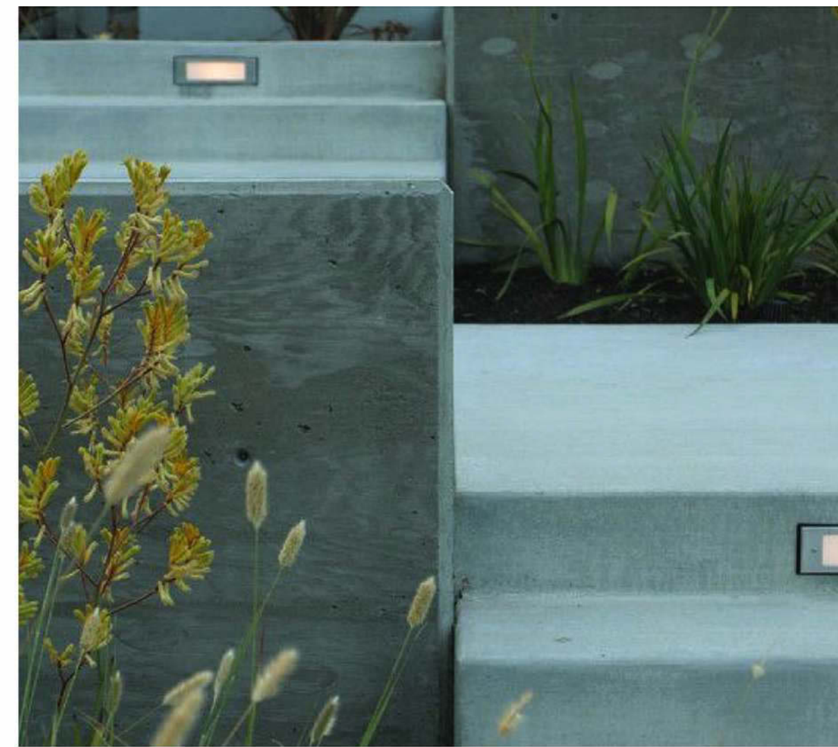
9 CIP CONCRETE STAIRS L6.0
