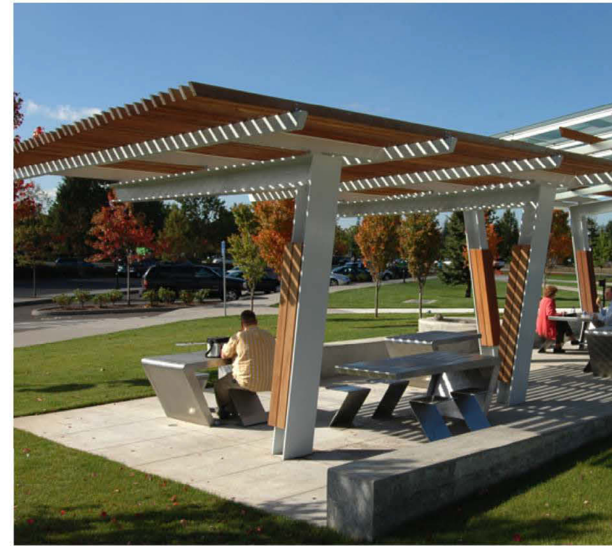
3 WOODEN TRELLIS WITH STEEL FRAME FOR SRW COMMUNAL AREA L6.1
