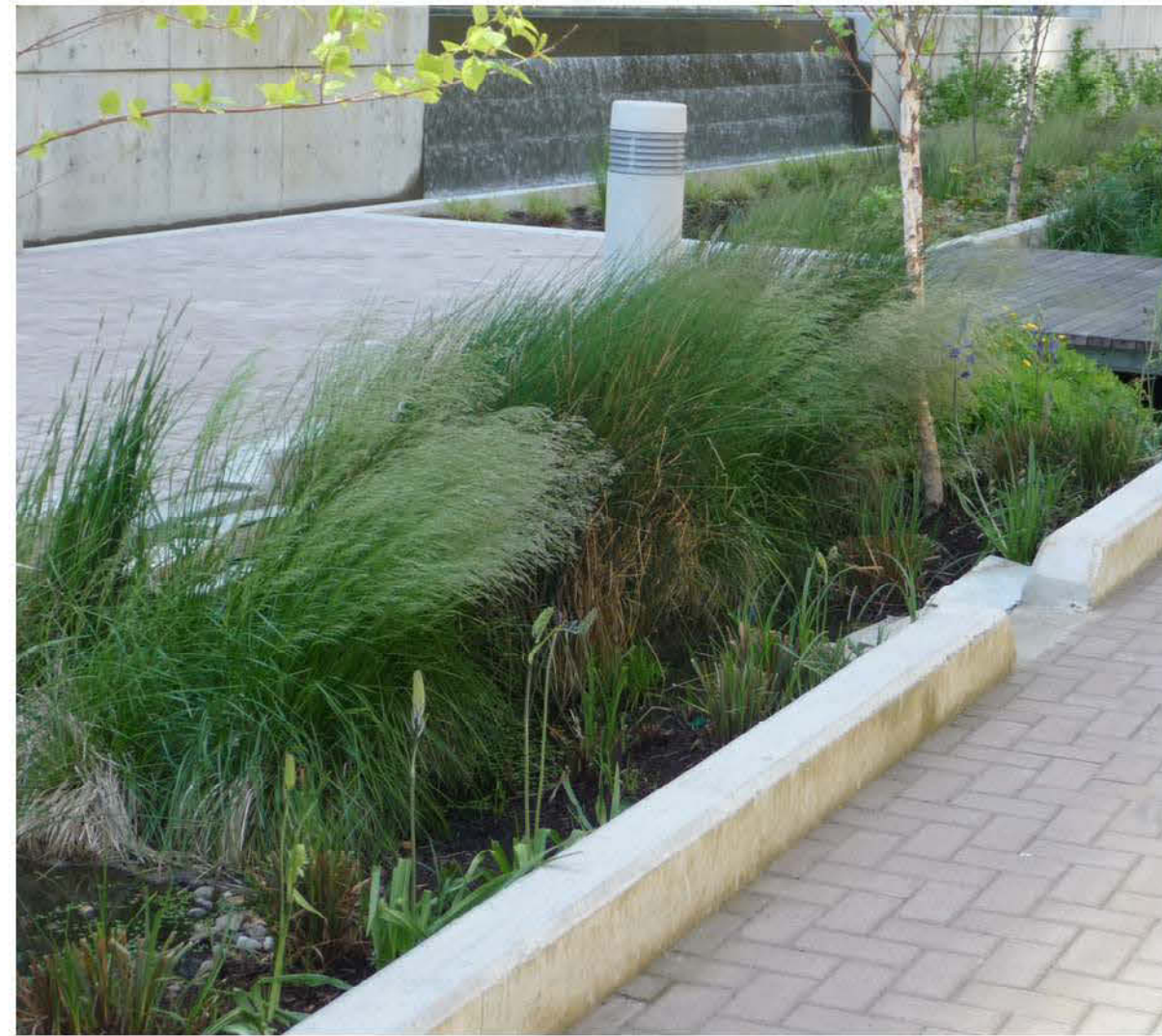
1 RAIN GARDEN WITH CONCRETE RETAINING WALL L6.1
