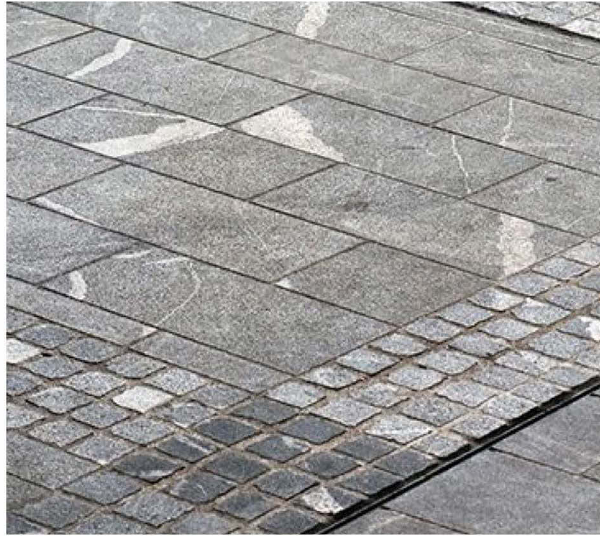
1 PAVING TYPE 1: ON/OFF SITE BANDING L6.0 Grey Granite Setts
