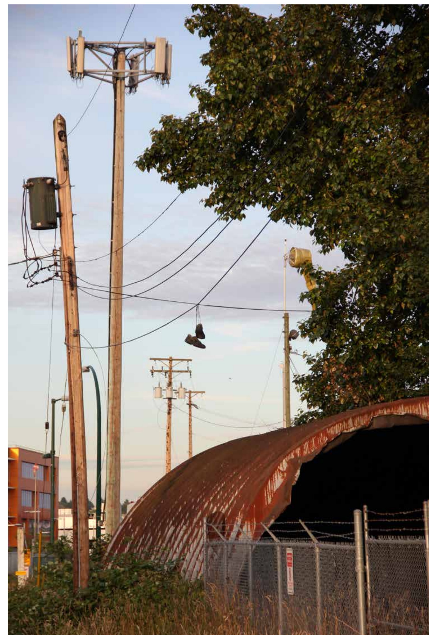
Hall on Northern Street
