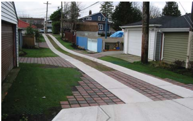
Laneway designed with natural stormwater management features.
