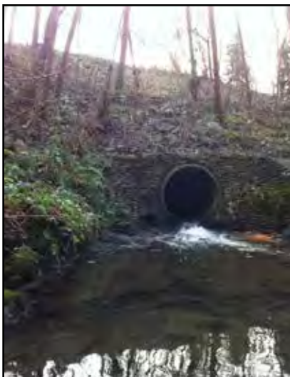
Culvert Outlet at 29th Avenue
