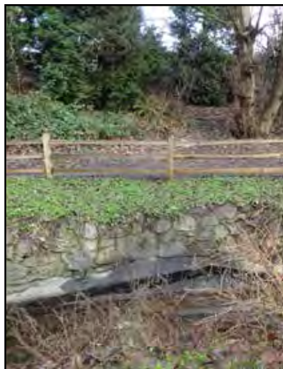
Existing Stream Bank Stabilization
