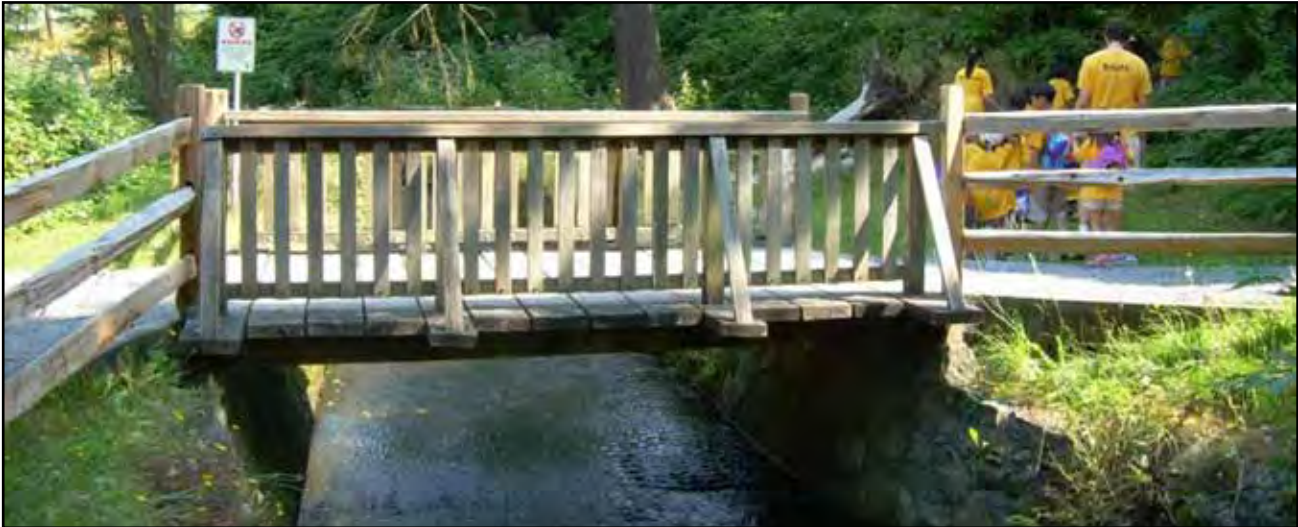
Foot Bridge over Still Creek in Renfrew Community Park
