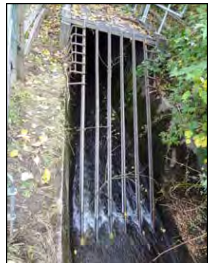
Debris Catcher where Still Creek Exits Renfrew Ravine
