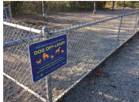
Example of a chain-link fence
