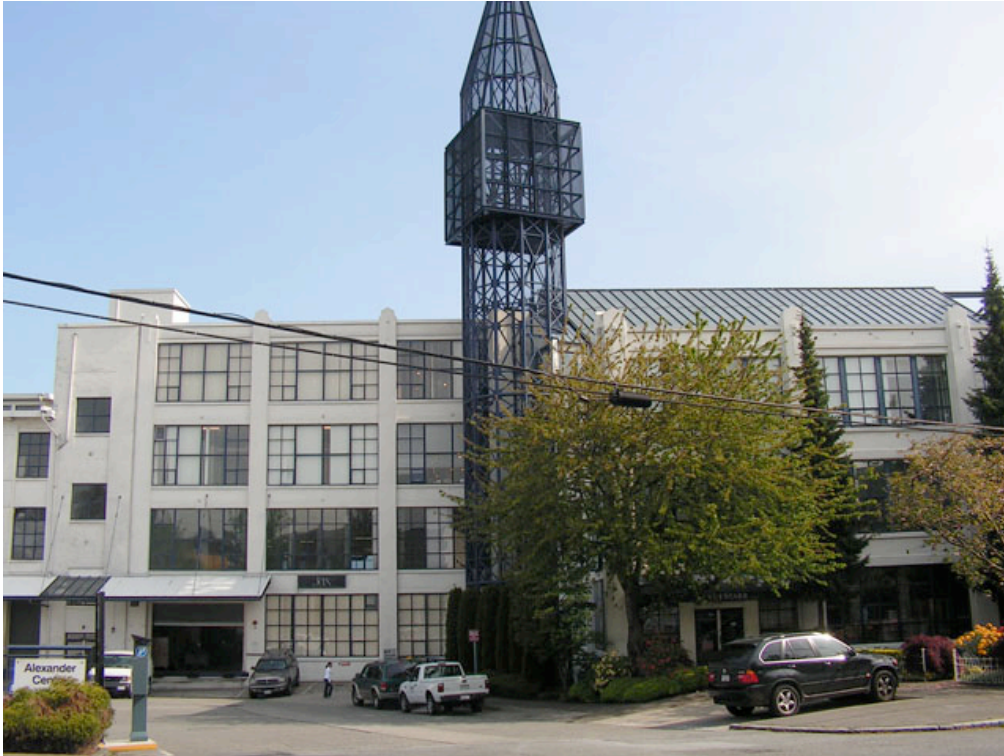
Source: Harris Consulting Inc.
