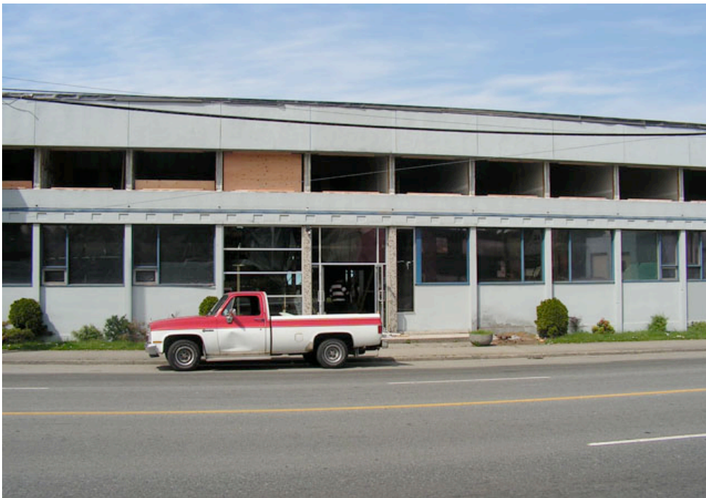
Source: Harris Consulting Inc.
