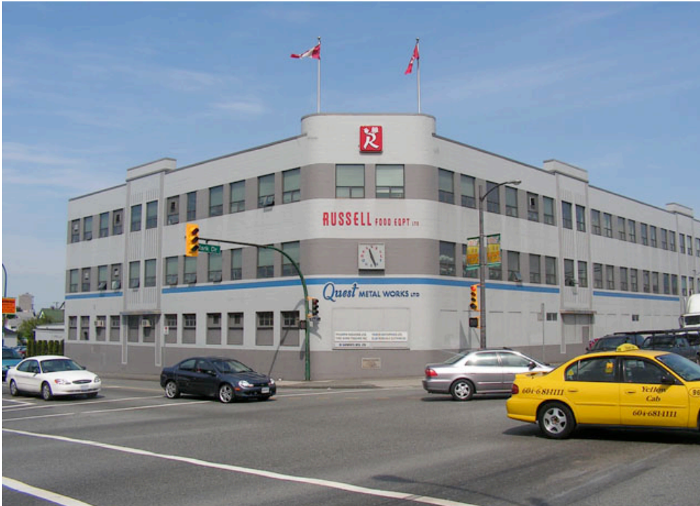
Source: Harris Consulting Inc.
