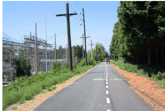
BC Hydro Substation Looking North
