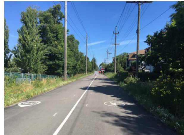
W 71st Looking North
