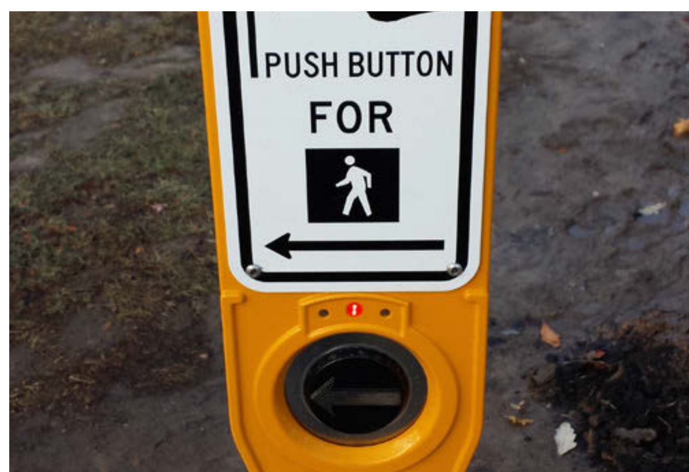
Accessible pedestrian signals
