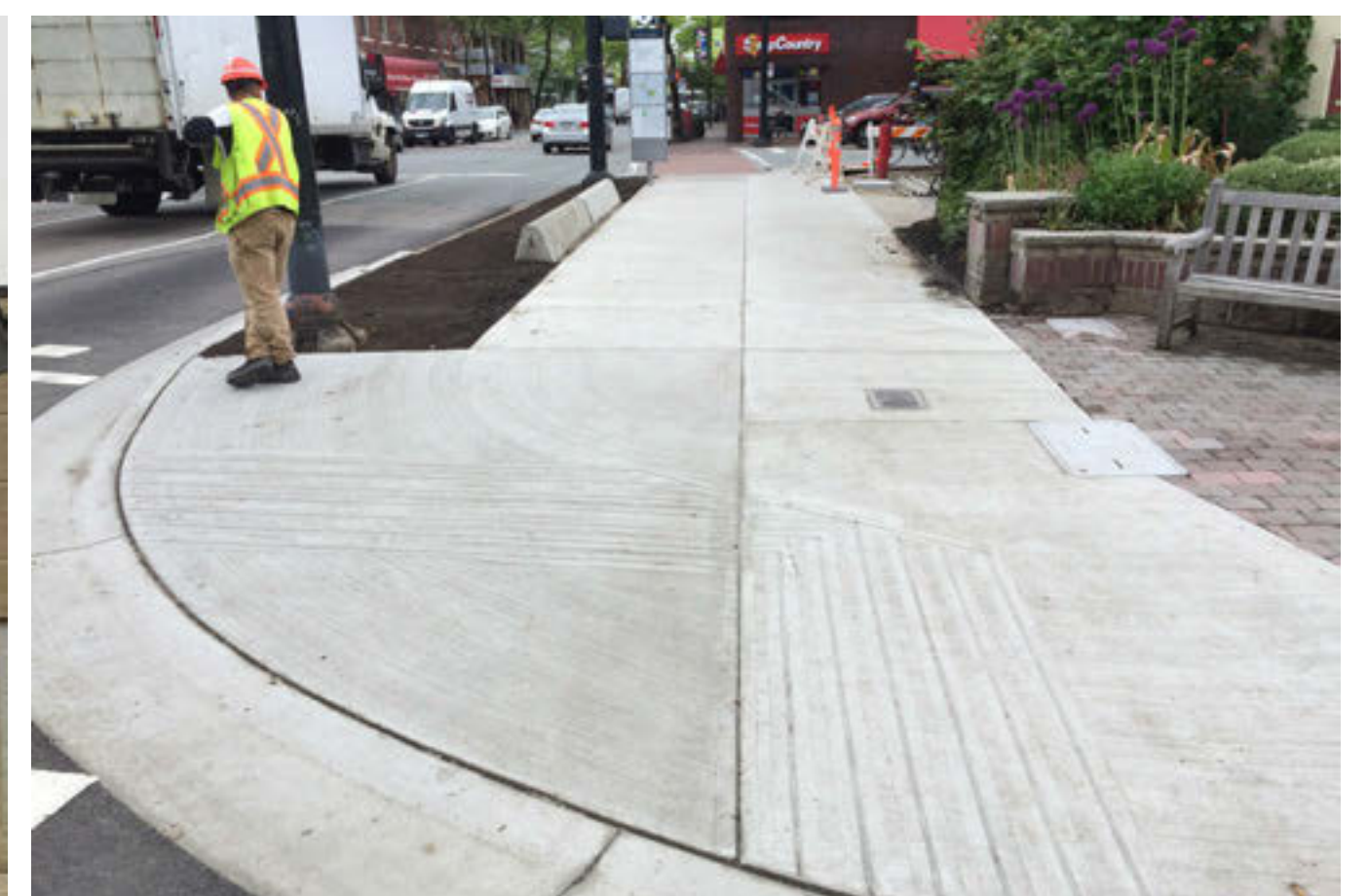
Curb ramps between sidewalk and street
