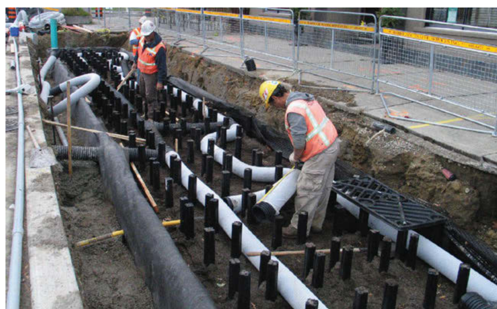
Rainwater detention in tree pits - Etobicoke ON (Image credit: Marco Clausen)
