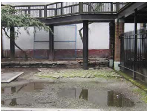
Pooling water, missing granite pavers
