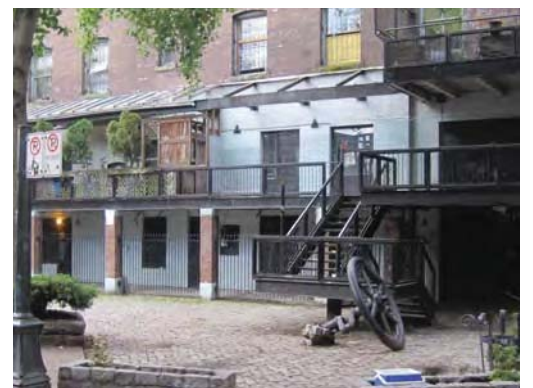
Staircase connecting the ground floor of Stanley New Fountain to Blood Alley Square
