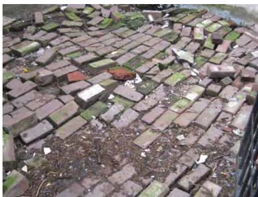
Uneven, disturbed red clay bricks
