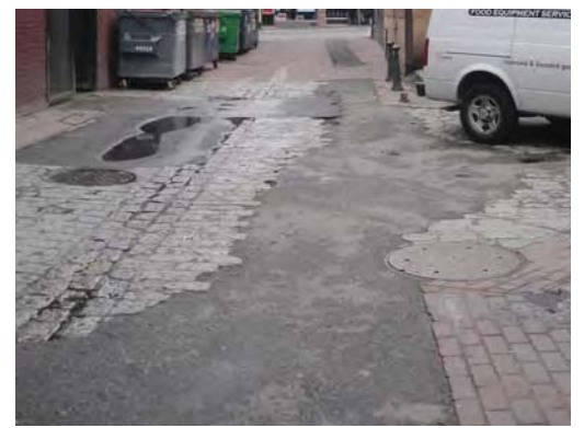
Asphalt repairs over granite and brick pavers
