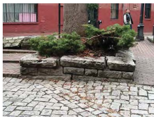
Red clay brick paver steps and ramp, granite block tree planters
