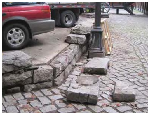
Dislodged granite block
