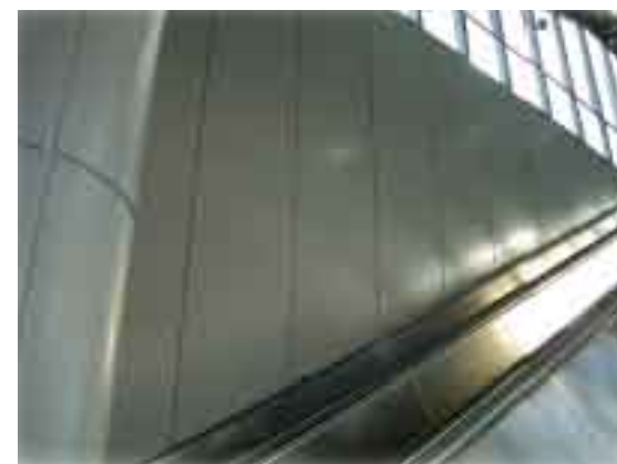
Sightlines between Commercial Drive and Broadway Stations are blocked by the Commercial Drive Station utility room and Shoppers Drug Mart building thereby inhibiting wayfinding between the two stations.
