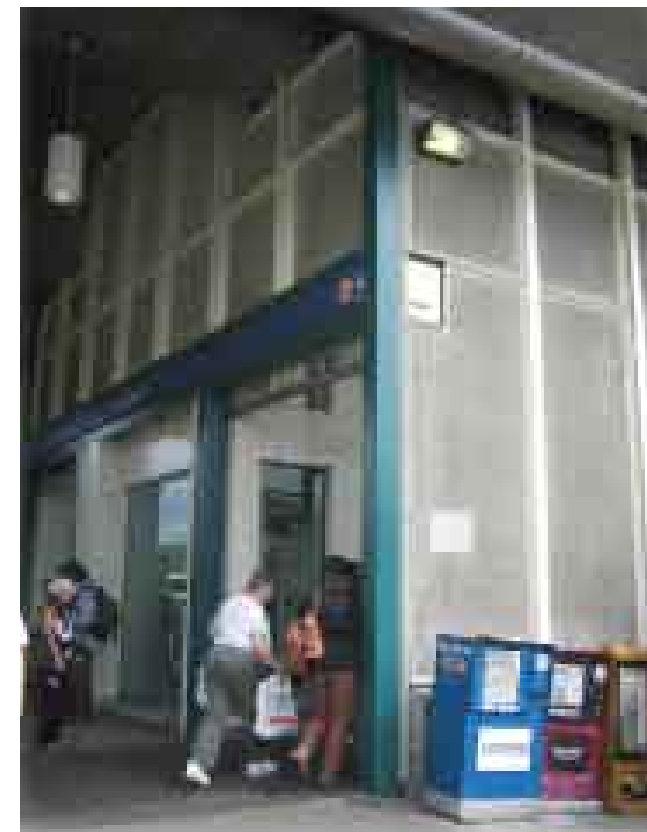
A single north entry to Broadway Station provides access to an elevator, escalator and stair system. At street level the elevator is a significant visual barrier to the station entrance.
