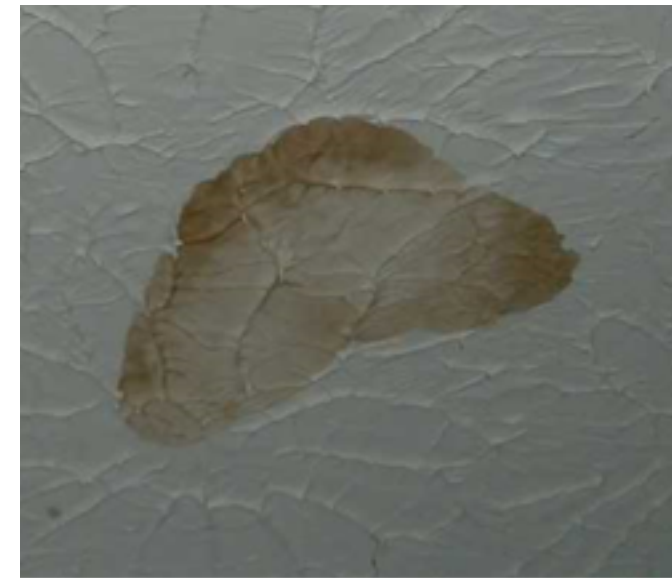
Evidence of Leaks
