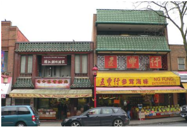
Vernacular buildings on the 200 block of East Pender c. mid 1970s
