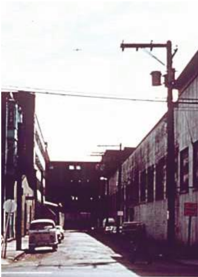
Shanghai Alley looking south, 1974 Vancouver Archives CVA 780-462
