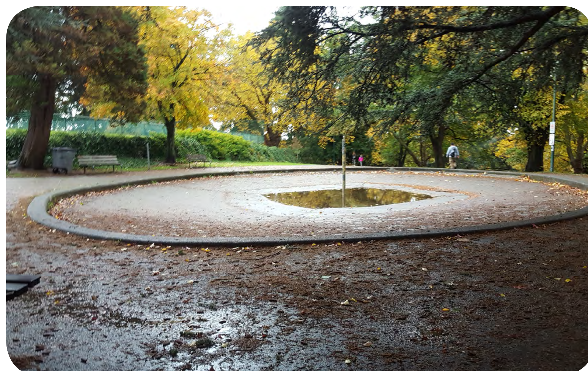
Decommissioned water pad
