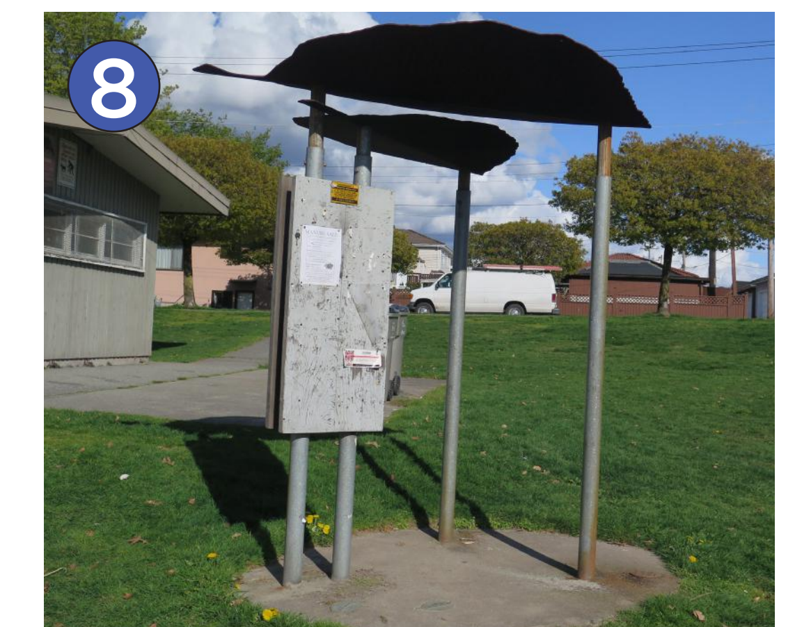
8 Signage in poor condition
