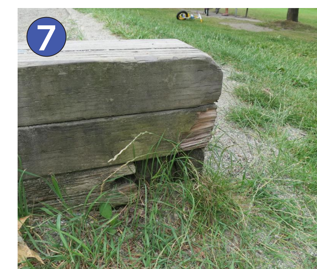
7 Worn site elements
