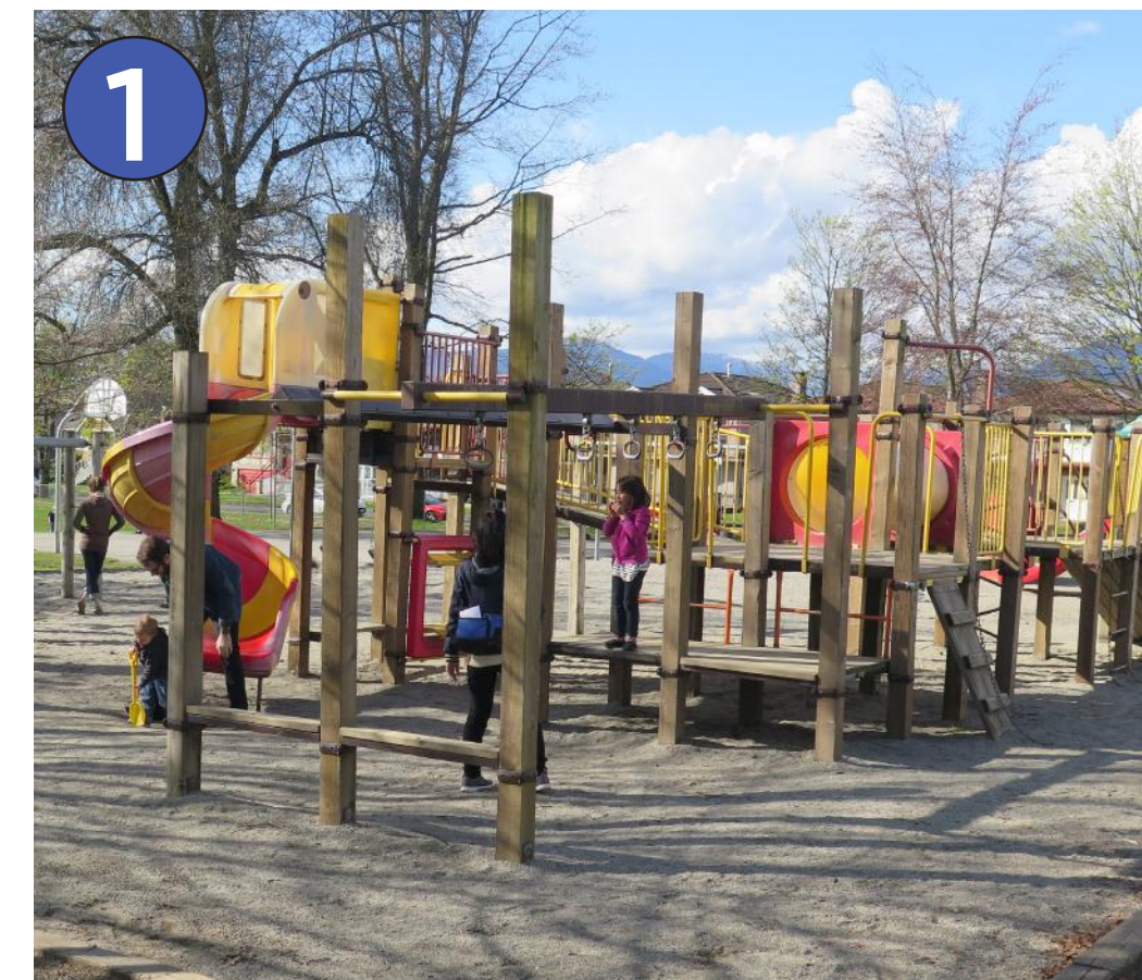
1 Playground equipment safety issues
