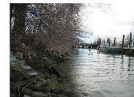
Concrete rubble along marine industrial use east of Fraser Street (C. Farland, March 2014)
