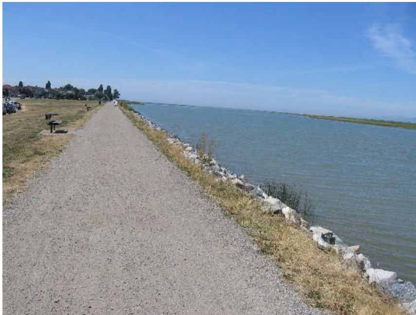
Middle Arm Dike, Richmond
