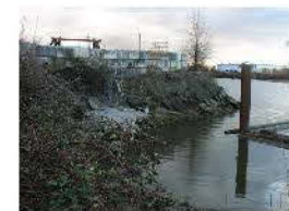
Gradually eroding bankline with lock-block wall about to be underlined (C.F. 2014)
