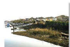
Debris flow from Corrington Street access at west end (S. Forstad, March 2014)
