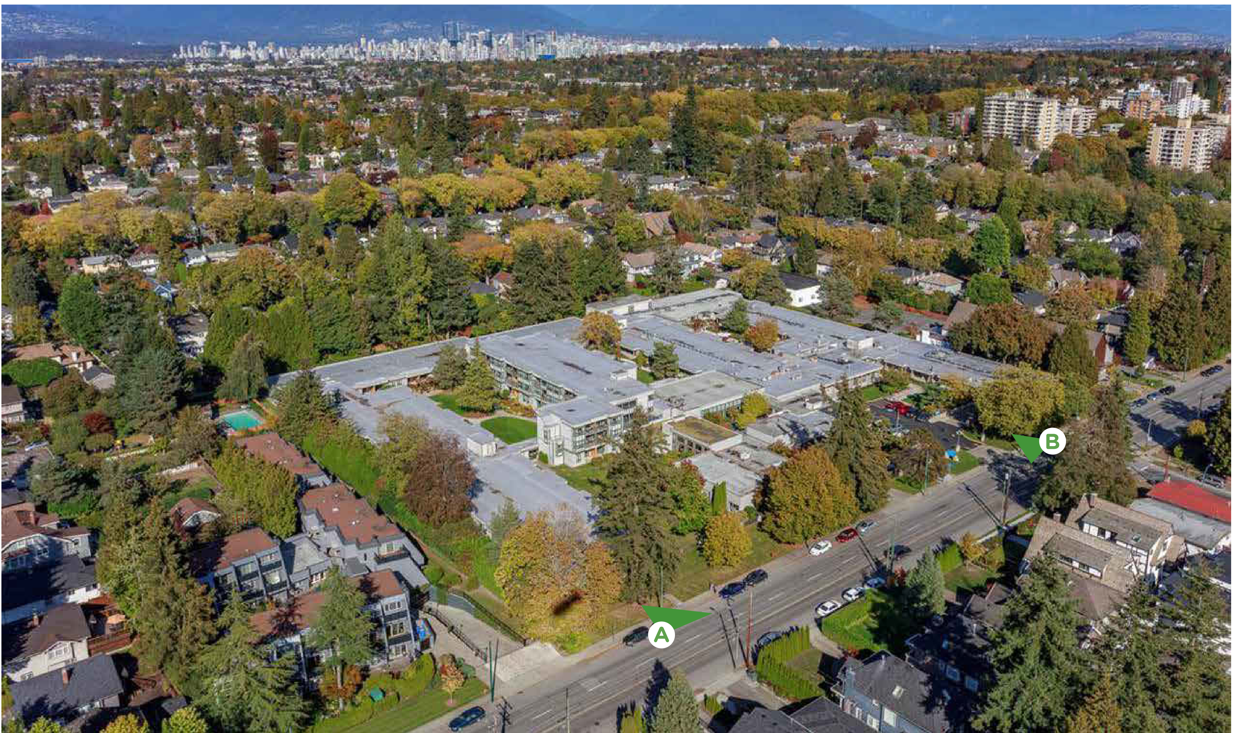
Aerial view of Crofton Manor looking northeast.
