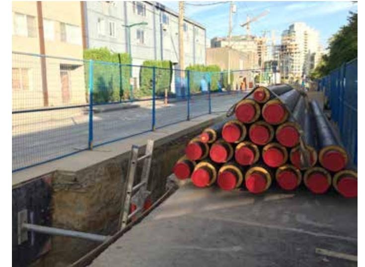
Some areas of the Flats are being integrated into the Southeast False Creek District Energy system
