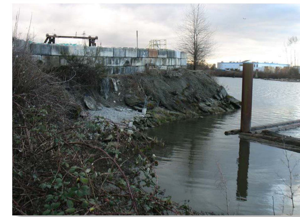
Gradually eroding bankline with lock-block wall about to be undermined (G.F. 2014)
