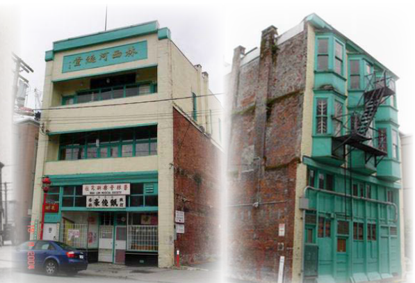
Carrall Street facade
