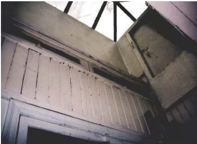
14 Skylight and roof access in Service Room
