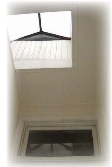
Skylight and high window (interior)
