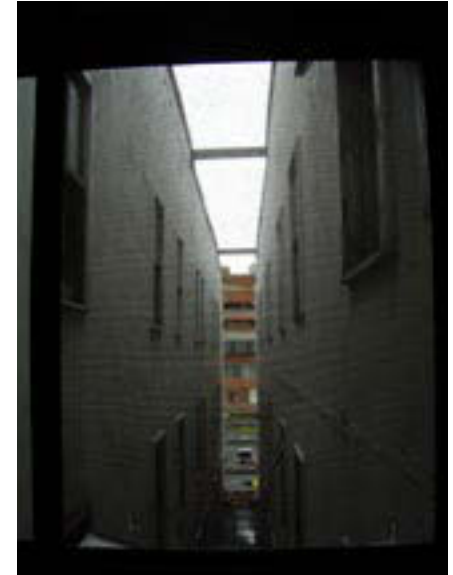
Typical lightwell looking from interior
