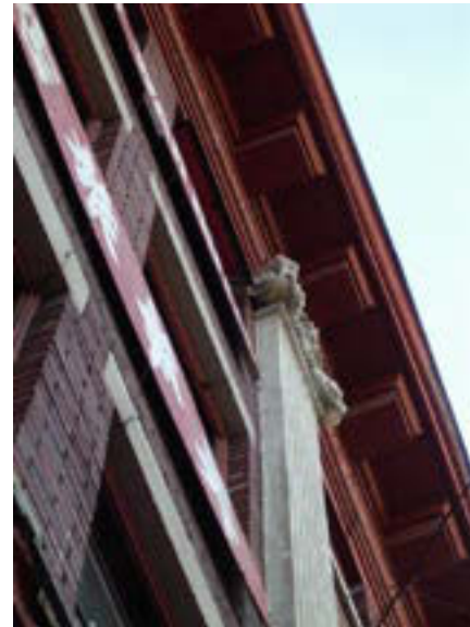
Details of cornice, dentil and column
