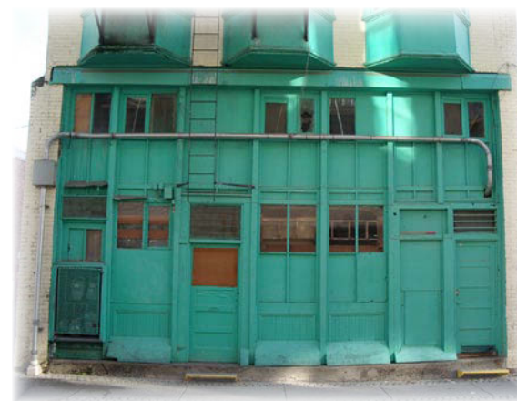
530 Shanghai Alley - Ground and Mezzanine Floor
