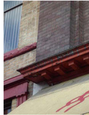
Cornice with dentil Details
