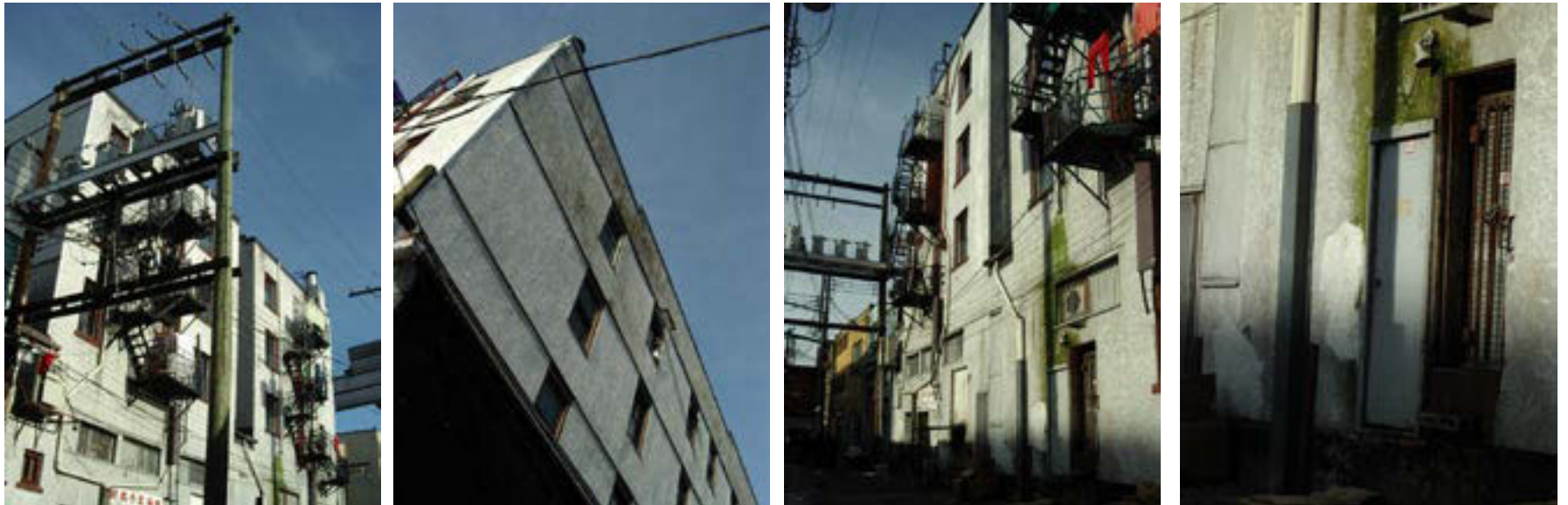
Photographs of rear facade of May Wah Hotel
