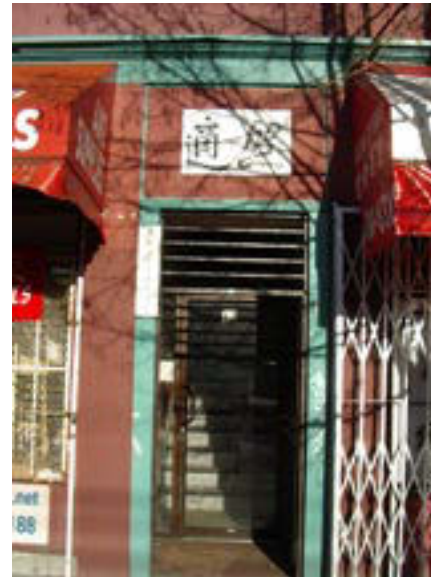
Street Entrance to 41-47 East Pender Street
