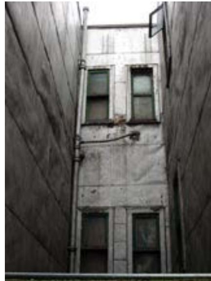
30-50 Market Alley: Interior lightwell on 2/F and 3/F
