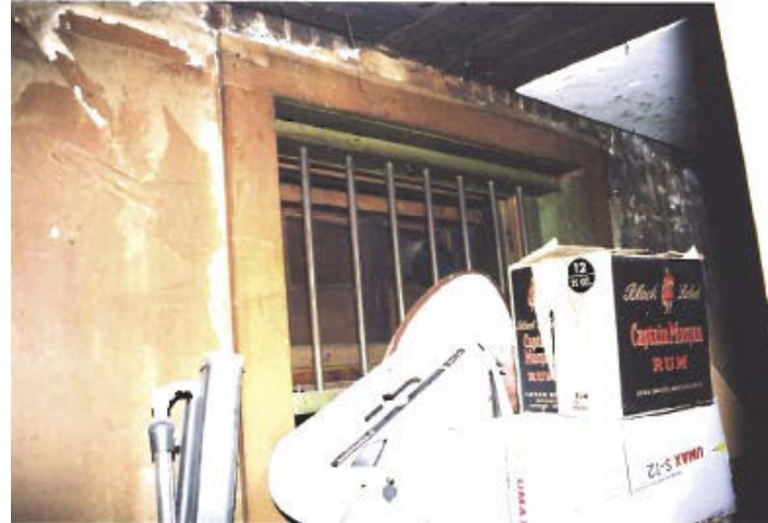
17 Blocked opening found in Mezzanine Floor of 525 Carrall Street
