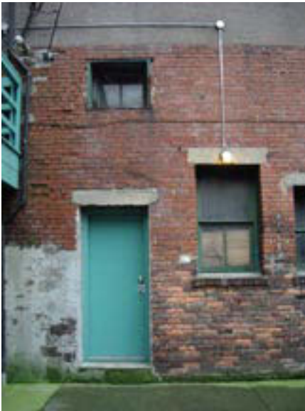
30-50 Market Alley: Ground Floor storage warehouse facing interior courtyard
