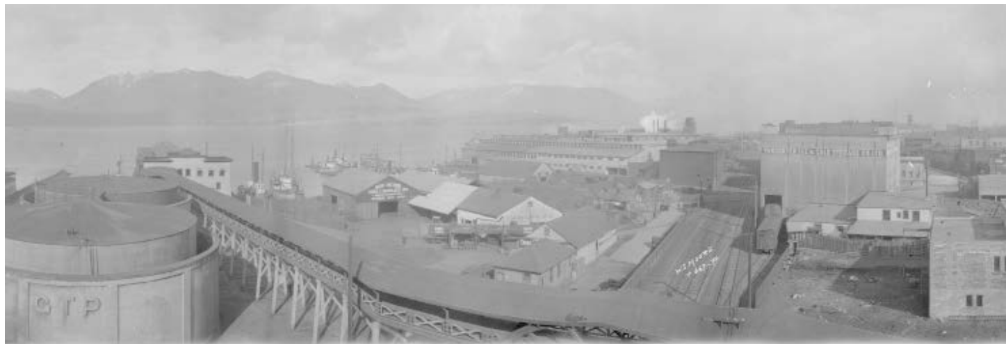
Waterfront with increase in industry. Grand Trunk Railway's wharves, fishing companies and the ice and cold storage facilities CVA PAN N229 - 1923
