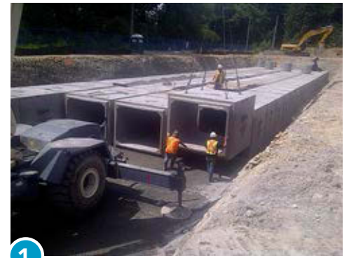
1 UBC Detention Tank Installation
