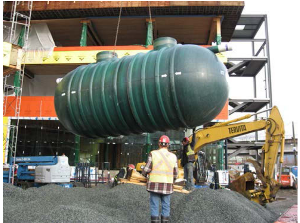
Detention Tank Installation, MEC Head Office
