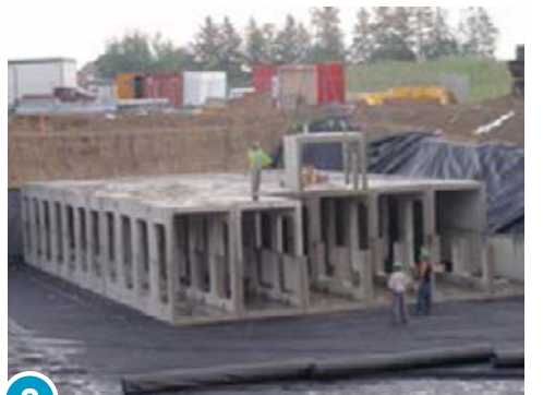
2 StormTrap Detention Installation (Photo credit: Sustainable Technologies Evaluation Program)
