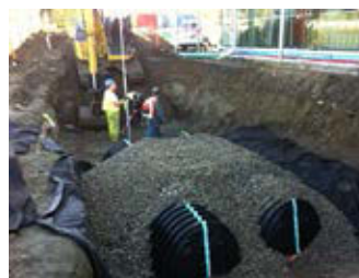
Infiltration Chamber Installation, MEC North Vancouver
