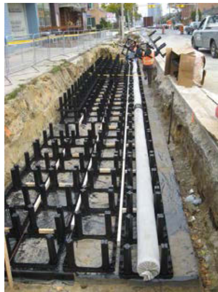
Perforated drain line is installed at the bottom of the 1st layer of Silva Cells and connected to the catch basin.
