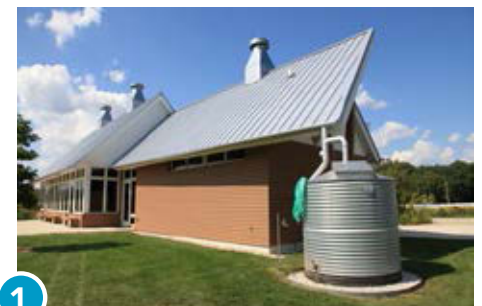
Above Ground Rainwater Harvesting System ( www.completeenergyuk.co.uk )
