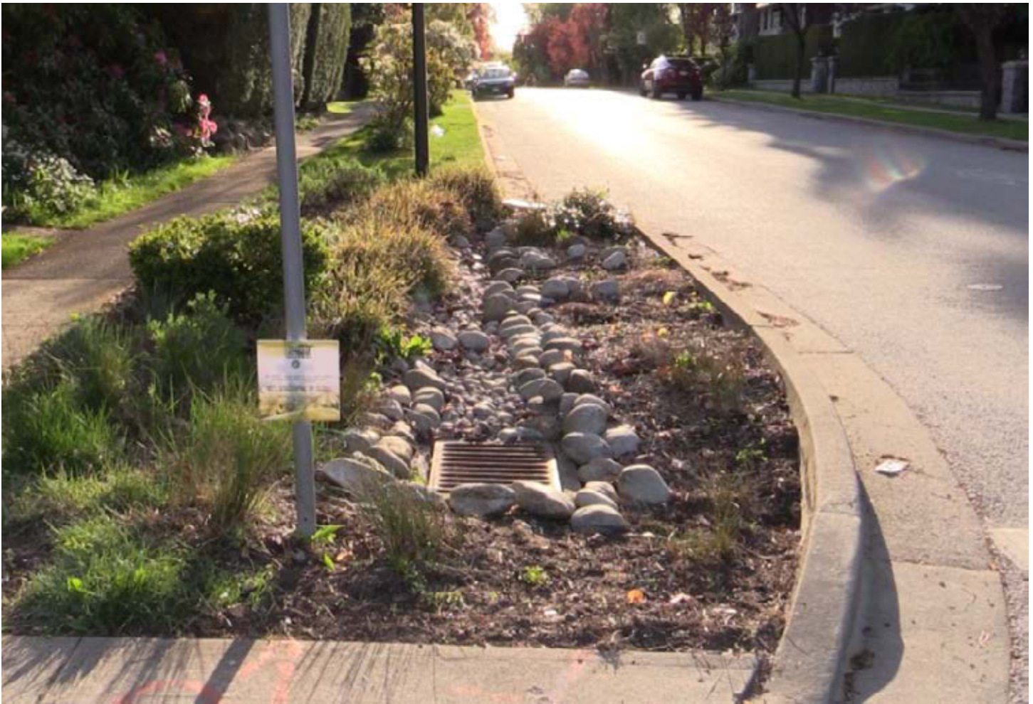
Stormwater Source Controls, like these infiltration bulges in Vancouver streets, are part of Climate Change Adaptation green infrastructure.
